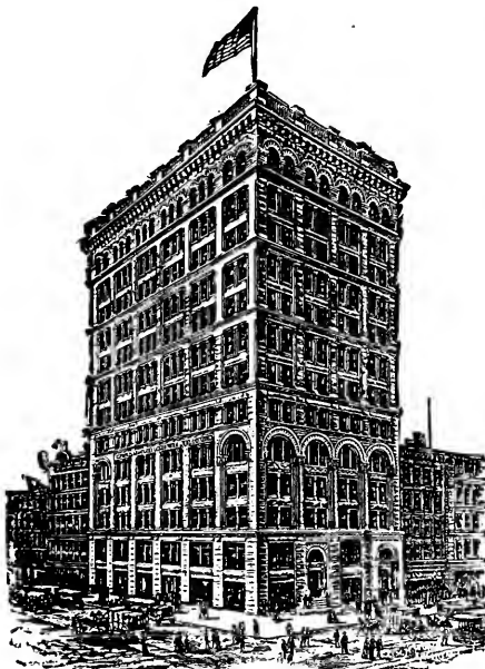
MUTUAL RESERVE BUILDING.
