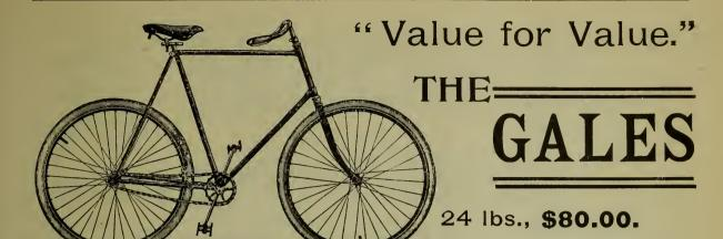
We offer you the best that can be obtained at any figure, and charge a reasonable price. The Gales is equal to any wheel on the market in quality, and is up to date in all features. Large balls in bearings, high frames, adjustable handle bars, dust-proof bearings, etc. In appearance it is a wheel to be proud of.
