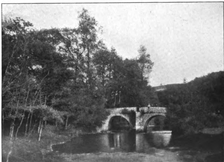
LODDISWELL MILL BRIDGE
