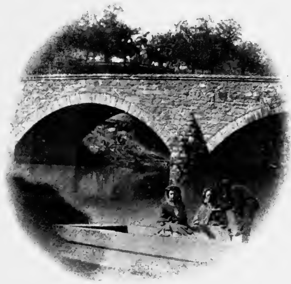
AT ANTIETAM BRIDGE
