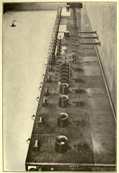
SWITCHBOARD CONNECTING ALL THE MOTORS IN A COLUMBIA, S. C., COTTON MILL OPERATED ENTIRELY BY ELECTRIC POWER.
