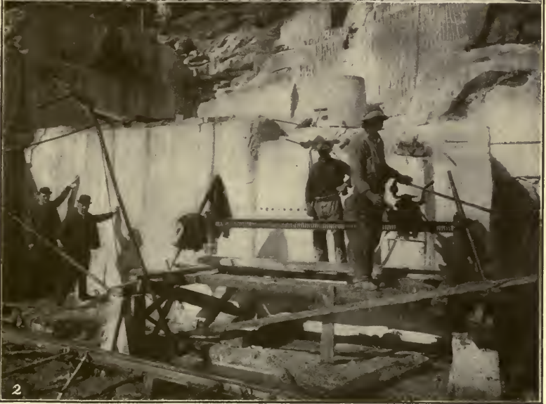
TWO VIEWS OF MARBLE QUARRY NEAR KNOXVILLE, TENN.
