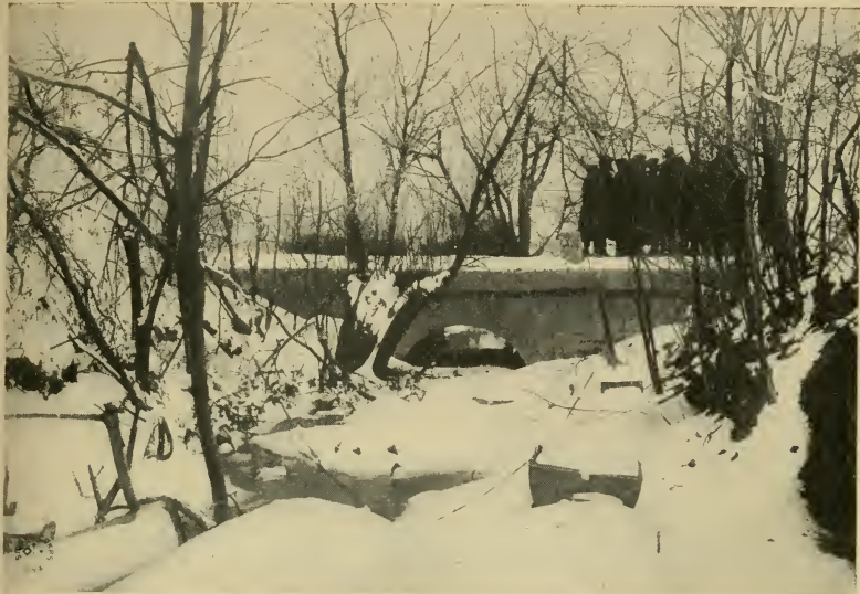
Culvert near "bloody angle," Junction St. Juvin-Sommerance Road
