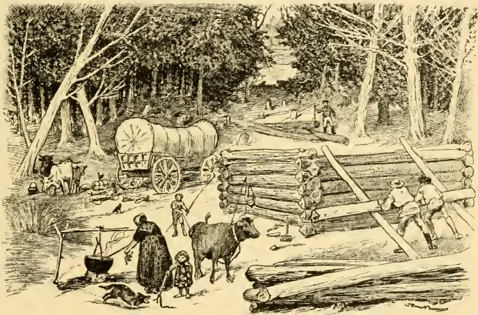
BUILDING A LOG HOUSE
