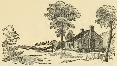
BIRTHPLACE OF WASHINGTON The site of the house is now marked by a monument.
