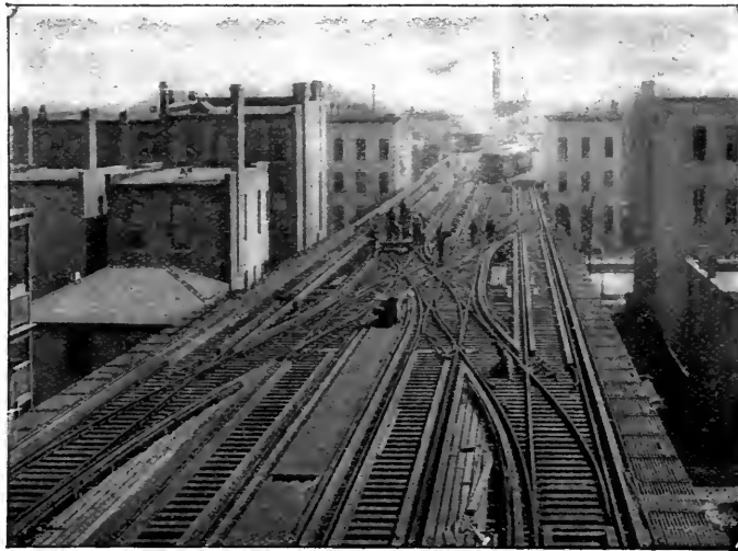
FIG. 345. CHICAGO ELEVATED ELECTRIC RAILWAY.
