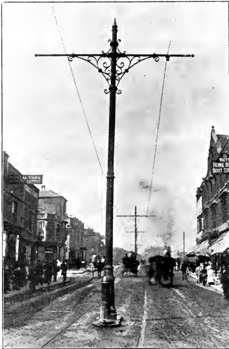
FIG. 390. CENTRE POLE CONSTRUCTION, LAURENCE HILL.
