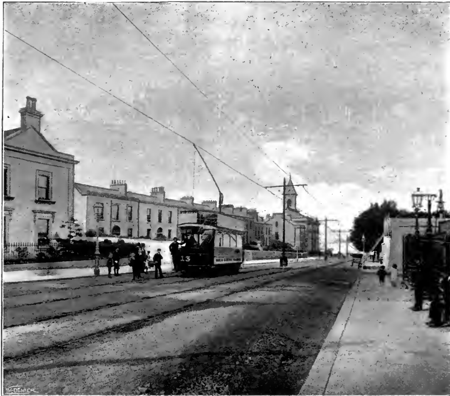
FIG. 353. CENTRE-POLE SYSTEM, DALKEY.
