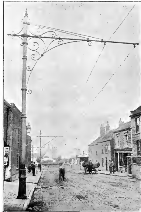
FIG. 391. 16-FT. BRACKET ARM AT ST. GEORGE.
