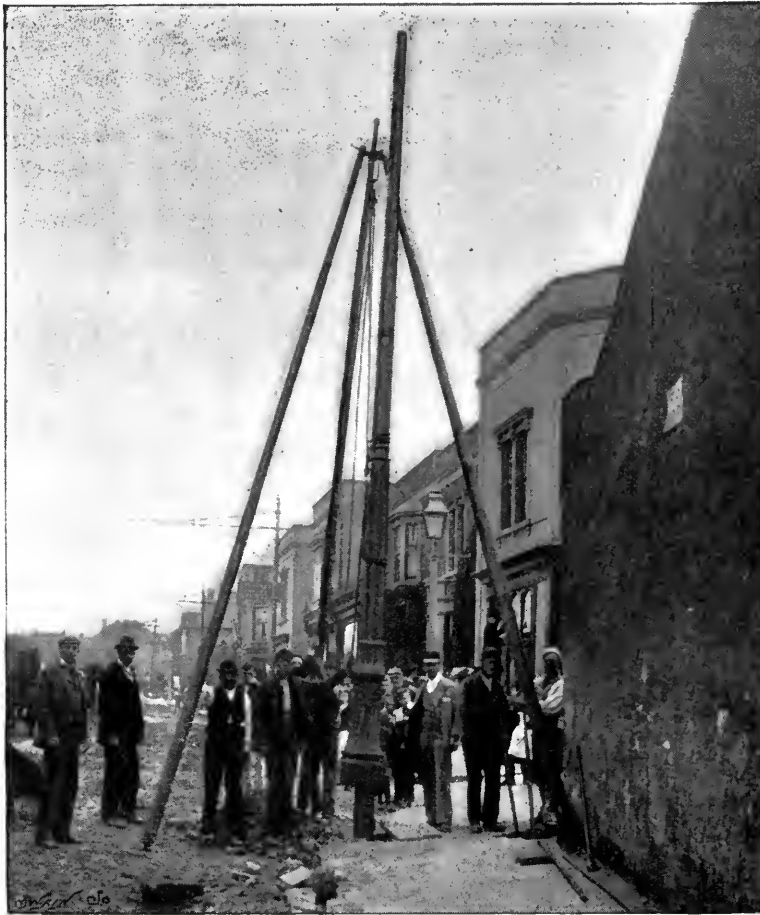
FIG. 137. PLANTING POLES ON THE BRISTOL ELECTRIC TRAMWAYS.
