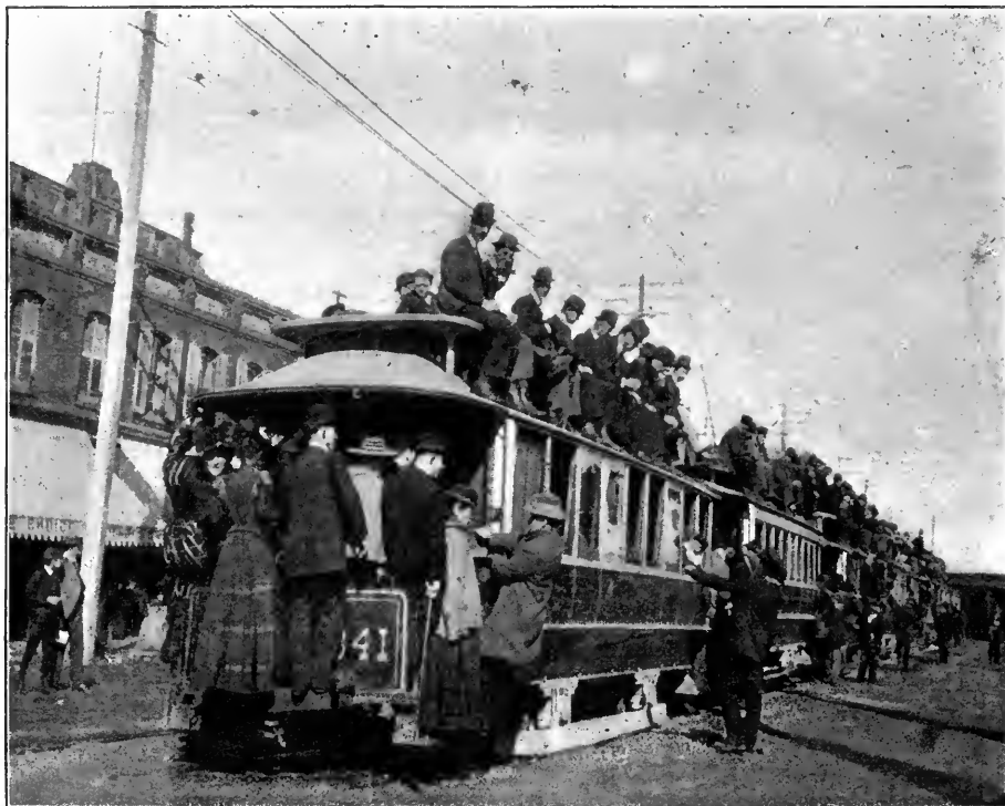
FIG. 218. TRAIN OF CABLE CARS AT CHICAGO, "CHICAGO DAY," WORLD'S FAIR.
