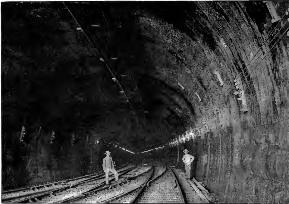
FIG. 329. INTERIOR OF BALTIMORE TUNNEL.
