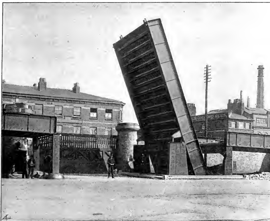
FIG. 403. OPENING BRIDGE ON LIVERPOOL OVERHEAD RAILWAY.
