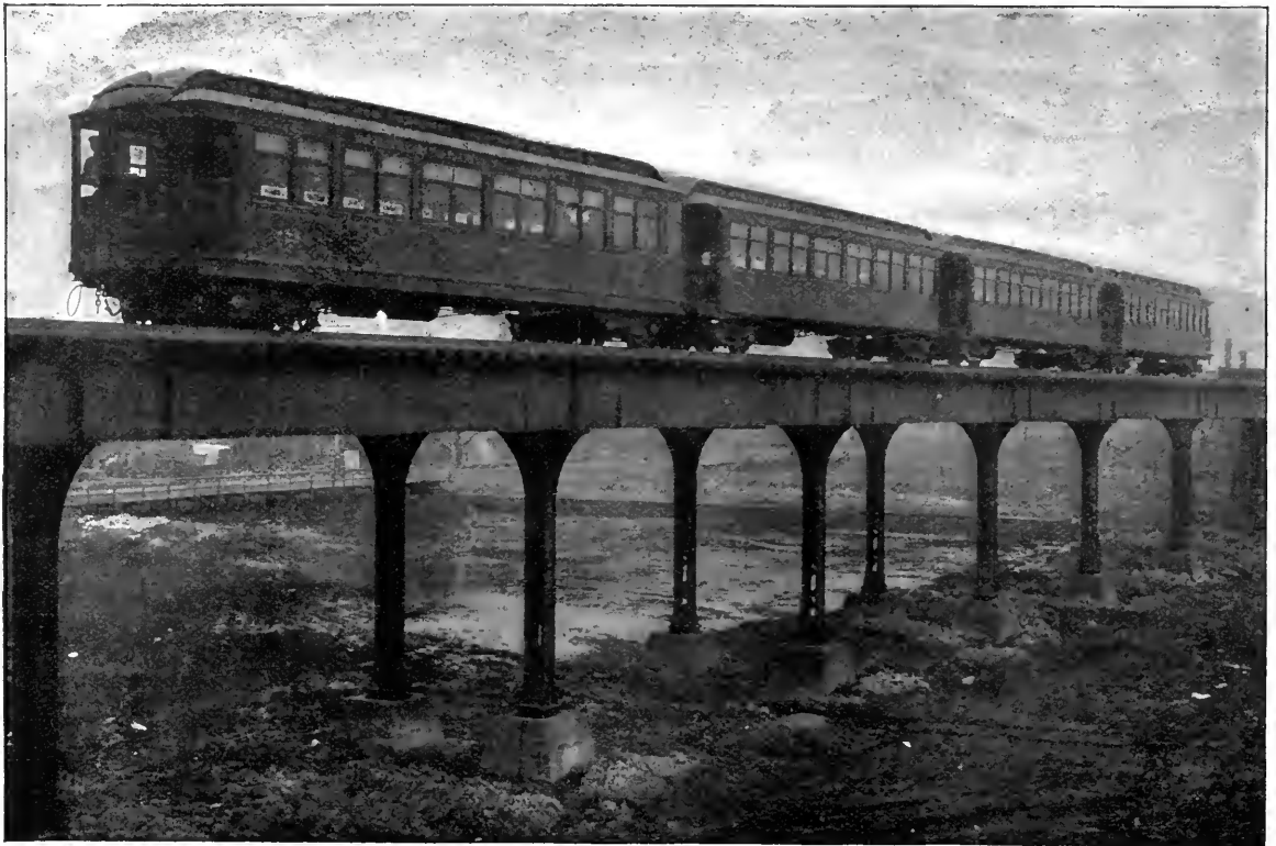
FIG. 344. CHICAGO ELEVATED ELECTRIC RAILWAY.
