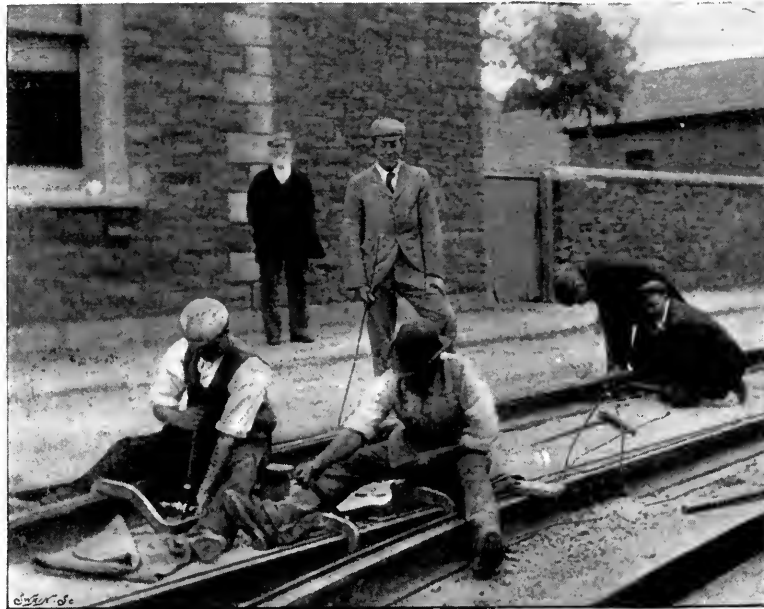
FIG. 50. DRILLING RAILS AND BONDING WITH "CHICAGO" BONDS AT BRISTOL, ENGLAND.
