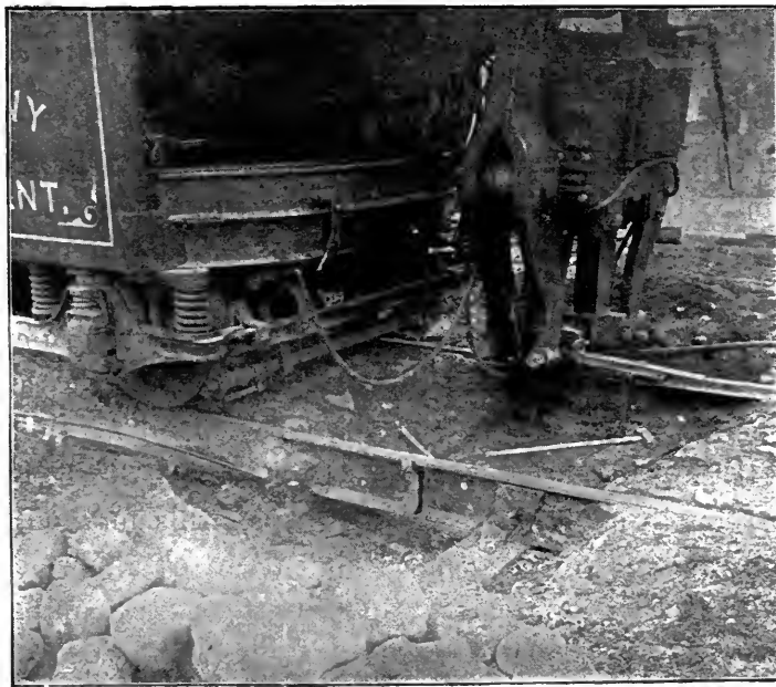
FIG. 58. RAIL WELDER.
