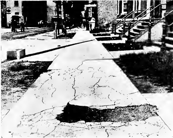
DISHONEST, SKIMPY WORK IN CONCRETE SIDEWALK CONSTRUCTION.
