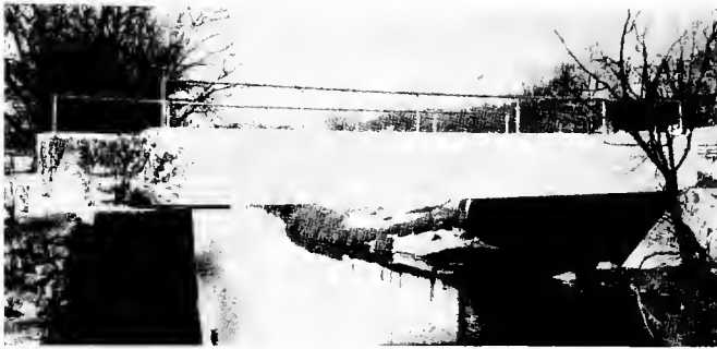
CONCRETE GIRDER HIGHWAY BRIDGE, BALTIMORE COUNTY, MD.
