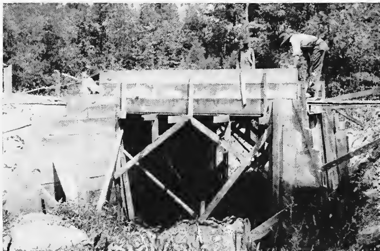
View during construction—Forms in place.
