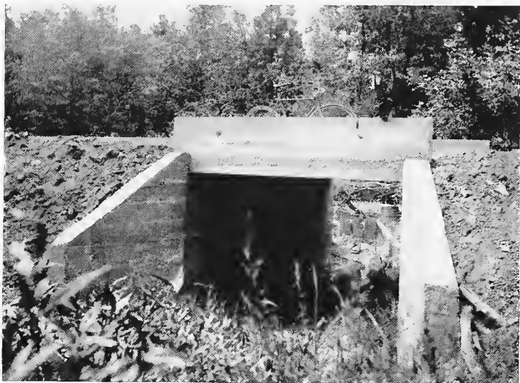
View after forms were removed and before dressing up.
