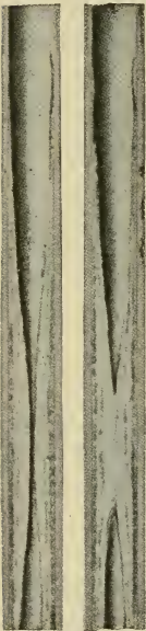
Pipes showing two months' scale formation in old-time water heater.
