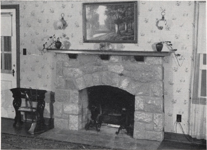
FIGURE 38.—This well-designed small stone fireplace was built in accordance with the principles given in this bulletin. It is a good heater and does not smoke. The jambs are wide enough to resist the thrust of the arch.
