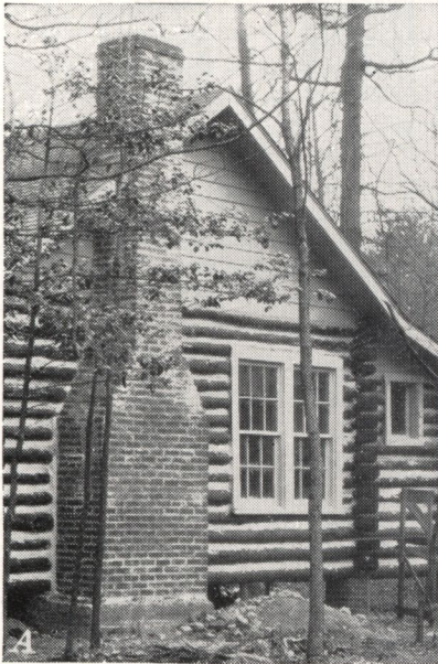
FIGURE 7.— A , A good foundation extending below the soil affected by frost. This chimney is well protected from ground moisture by the concrete carried above the surface; B , an insecure foundation. Supporting a chimney in this manner is a dangerous practice.
