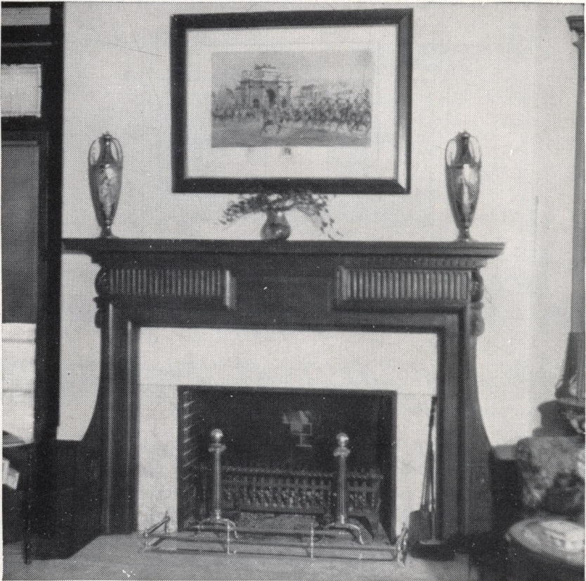
FIGURE 37.—Grates of this type are commonly used in fireplaces for burning coal or coke. This one has a metal back and ends and is only set in to permit proper circulation of air around it.
