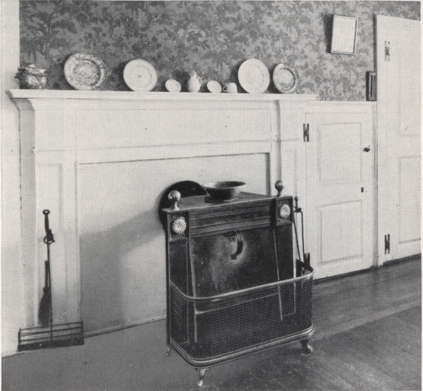
FIGURE 19.—In 1744 Franklin promoted a metal fireplace of this type to be set out into a room. These are known as Franklin stoves and sometimes are equipped with andirons for burning wood or a grate for burning coal. The metal blower, shown in front of the opening was used with grates and set in place when starting the draft and then removed so that the cheery heat of glowing coals could be enjoyed. At one time this type of stove was highly thought of because it threw out more heat than the built-in fireplace. A few manufacturers specialize in Franklin stoves because of the present-day demand.
