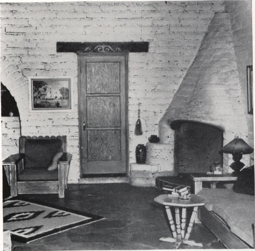
FIGURE 32.—An adobe fireplace of the Mexican-Indian type commonly built in the Southwestern States, especially when the house walls are of adobe. The logs are stood up, leaning against the back of the grate, in order to secure a high-licking flame.
