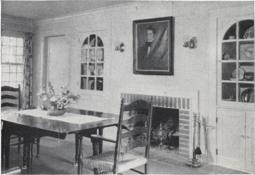
FIGURE 31.—This 36-inch-wide fireplace does not seem too large for the small room, but its size would have been accentuated by the use of a mantel.
