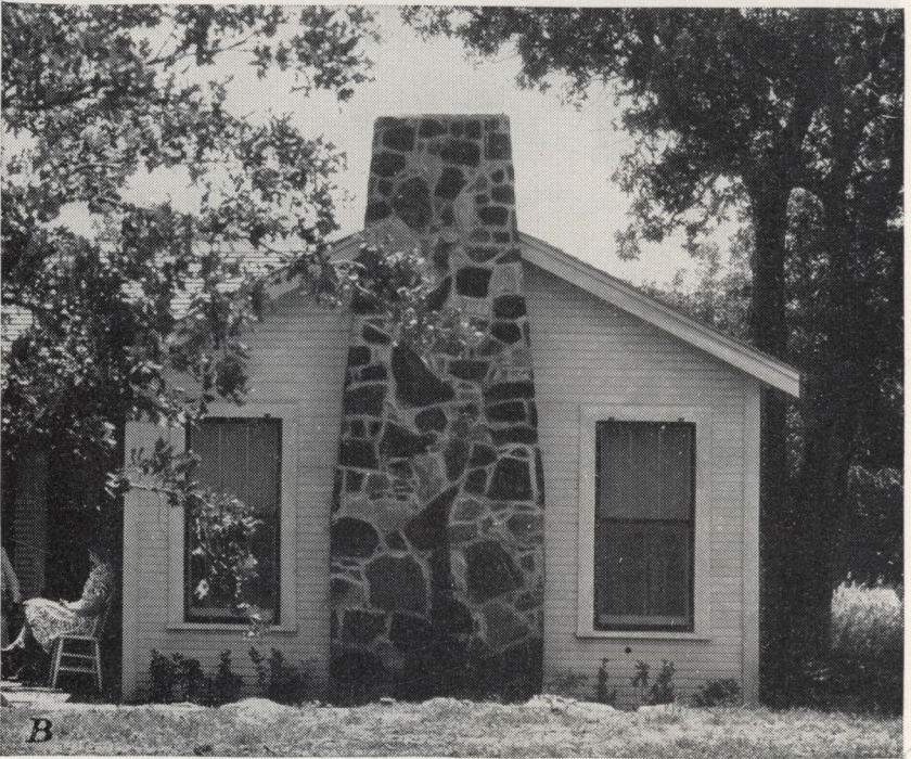
FIGURE 5.—Two pleasingly designed fireplace chimneys that fit into their surroundings. A , This chimney stands in the clear and should provide a good draft; B , a chimney under overhanging trees is likely to backdraft. Contrast the appearance of these two chimneys with that of figure 3.
