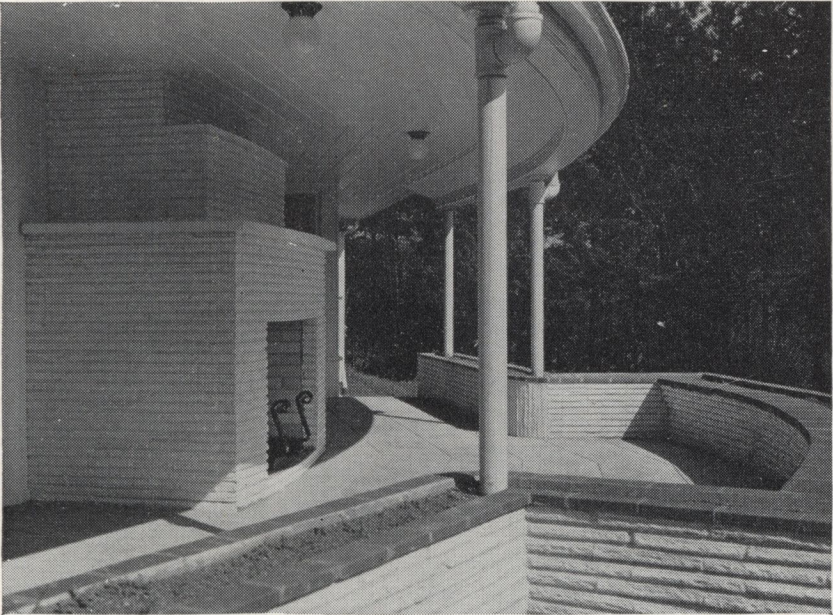
FIGURE 41.—An outdoor fireplace built back of an inside fireplace and opening onto a paved terrace provides comfort in early fall.
