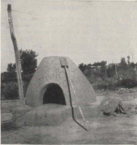
FIGURE 44.—This Dutch oven of adobe bricks is a type very common in the States along the Mexican border. It is called an orño and is usually built a short distance from the kitchen door.
