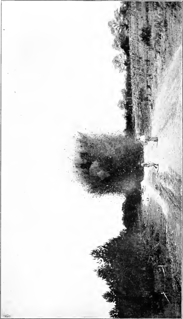
GRADING A ROAD—THE BLAST
