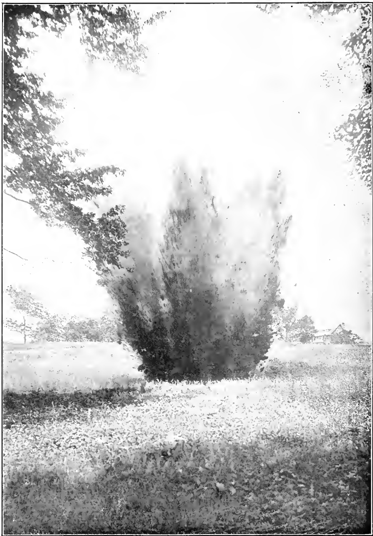
BLASTING A BOULDER
