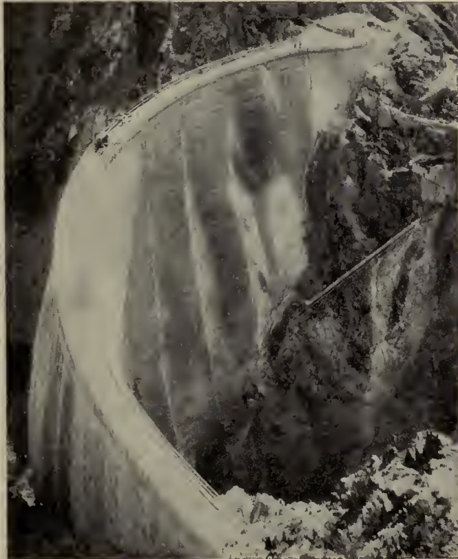
While a Dam Is Being Built the Course of the River is Changed—We See Here How the Finished Dam Looks Before the Water is Turned Back
