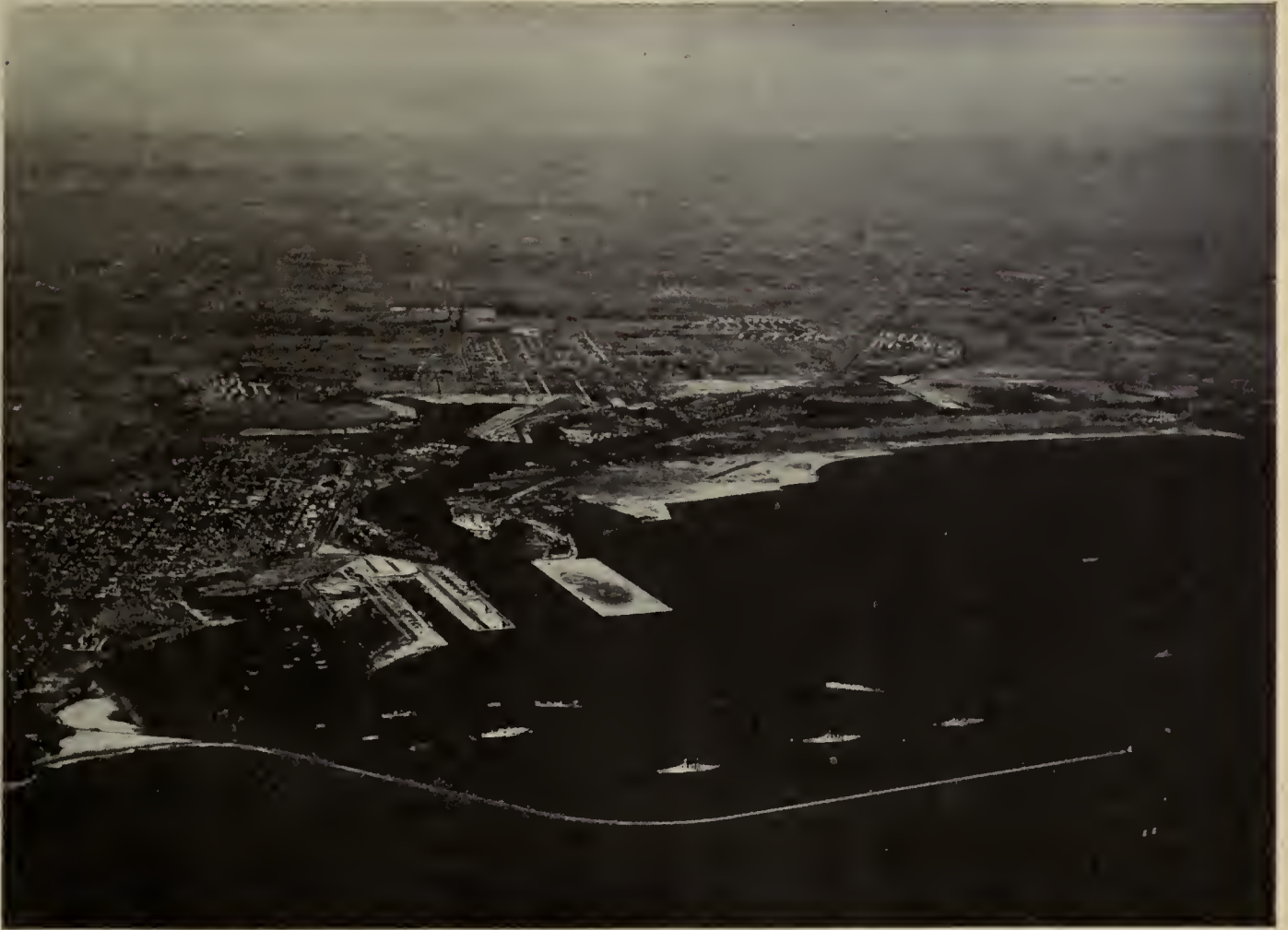
Airview of Los Angeles Harbor—Warships in Foreground
