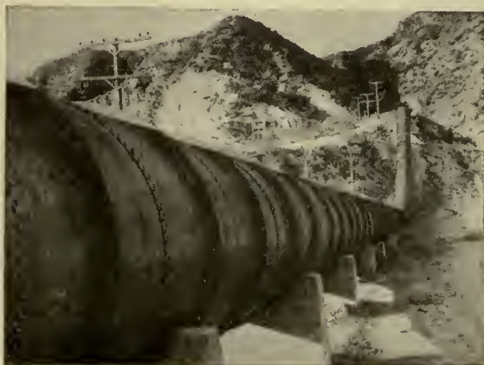
Huge Pipes Carry the Water
