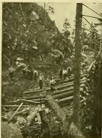
Mountain road building, Danby
