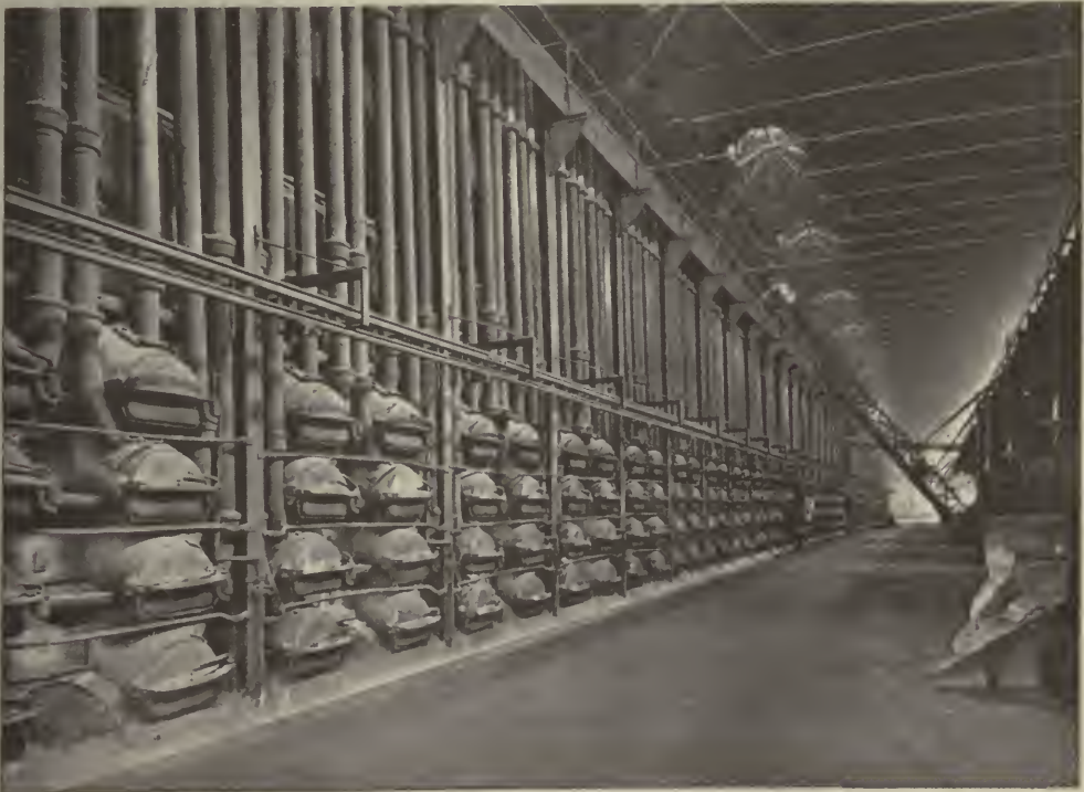
INCLINED RETORT HOUSE. KENSAL GREEN.
