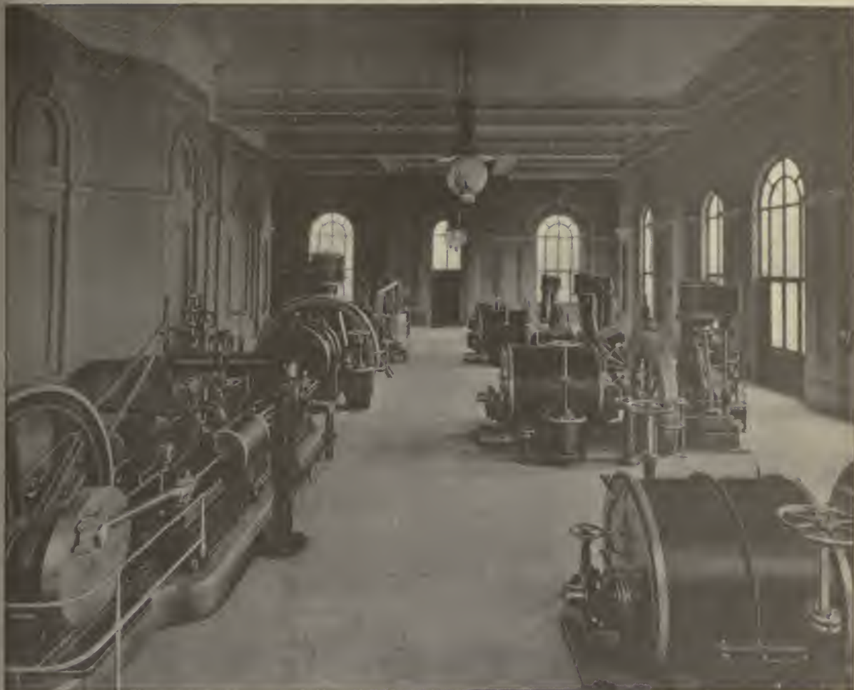
GAS PUMPING HOUSE, BROMLEY.
