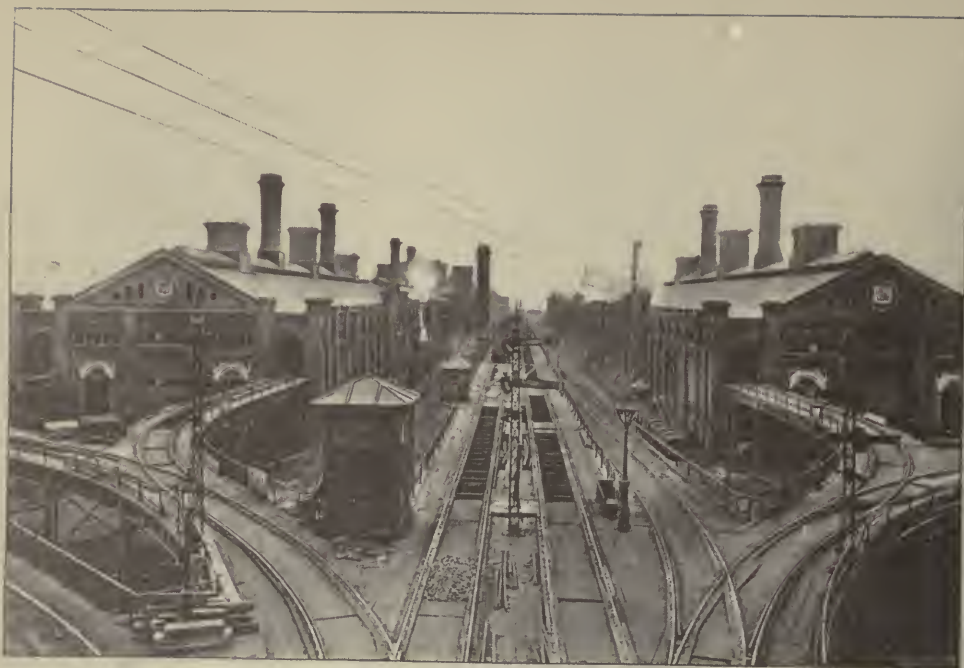
VIADUCT AND RETORT HOUSES, BECKTON.
