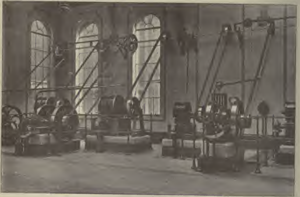
PRESSURE-RAISING PUMPS, WESTMINSTER.
