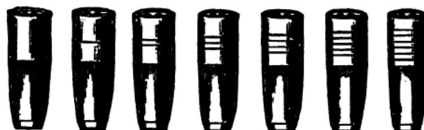
PATENT UNION-JET BURNERS, WITH PLUG SOCKETS, FOR SCOTCH CANNEL COAL GAS.
