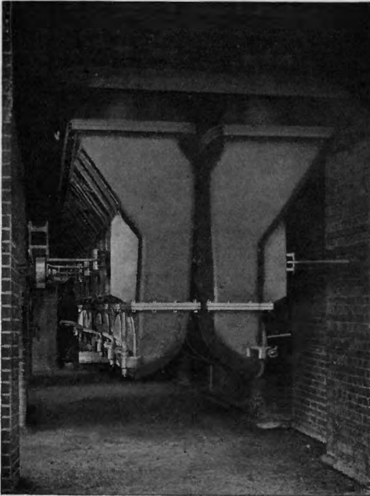
FIG. 12.—Glover-West coke chambers: Side view.
