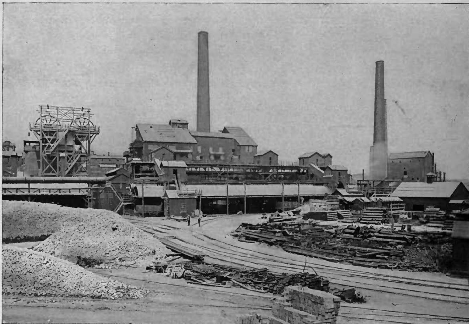
VIEW IN MESSRS. BRUNNER, MOND & CO.'S WORKS AT NORTHWICH, CHESHIRE, ENGLAND, SHOWING THE MOND GAS PLANT.
