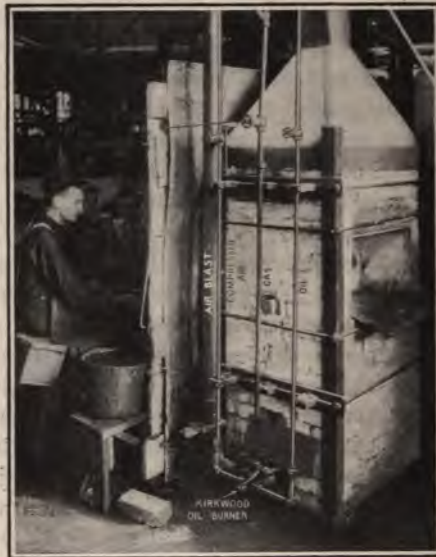
Fig. 57. Kirkwood Burners in "Glory Hole" at Heinz Bottle Works.
