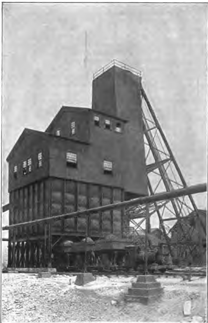
FIG. 10. HEAD-FRAME AND COAL BIN AT OLIVER NO. 3 PLANT
