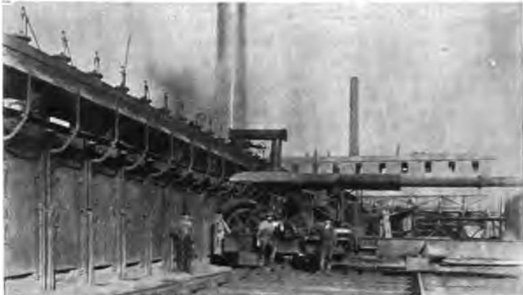
FIG. 21 (b). VIEW OF RAM AND FRONT OF OVENS
