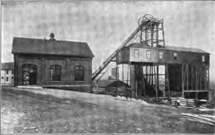
FIG. 8. HEAD-FRAME AND ENGINE HOUSE, PLANT No. 1, OLIVER COKE WORKS, REDSTONE JUNCTION, PENNSYLVANIA
