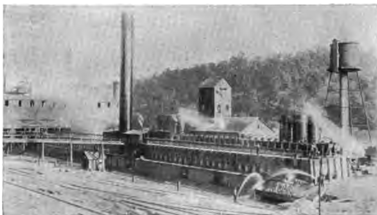
FIG. 21 (a). VIEW OF REAR END OF SEMET-SOLVAY COKE PLANT AT DUNBAR, PENNSYLVANIA
