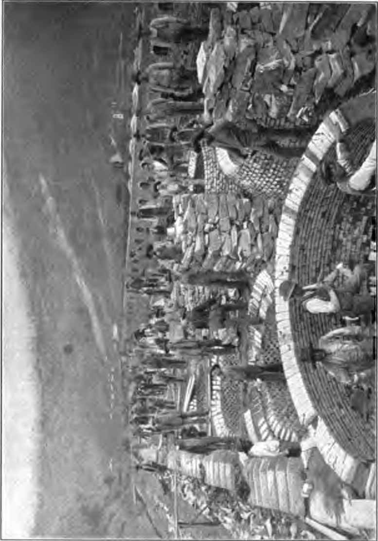
FIG. 9. CONSTRUCTING BEEHIVE OVENS
