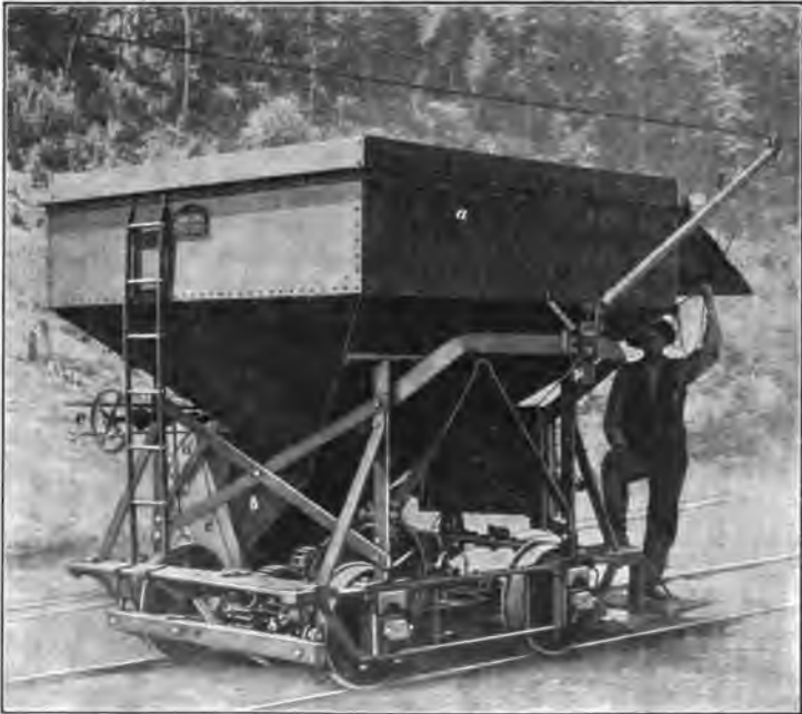
FIG. 1. ELECTRIC COKE LARRY
