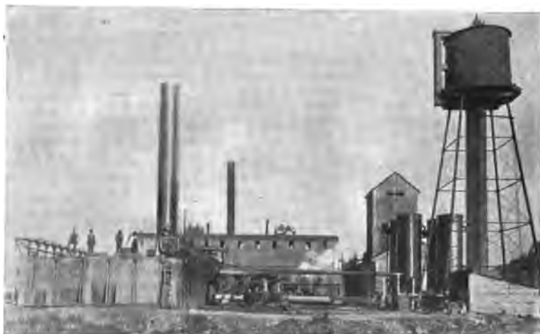
FIG. 21 (c). VIEW SHOWING ARRANGEMENT OF BY-PRODUCT APPARATUS
