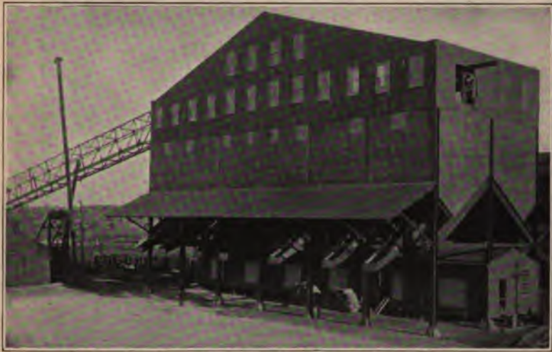
FIG. 135.—Coke-screening plant at Everett, Mass.
