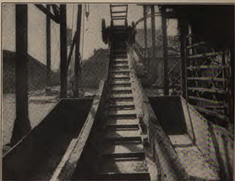
FIG. 132.—Delivery end of De Brouwer conveyor at Providence, R. I.
