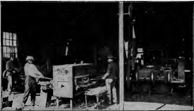
Fig. 198. Furnace serving two bolt headers.
