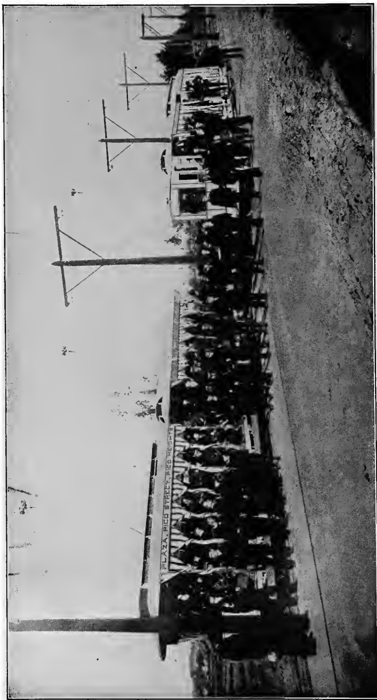
Fig. 1. The first electric locomotive built in the United States, drawing two trailers; also the first overhead wire system for trolley cars. Constructed in Los Angeles, California, in 1886.
