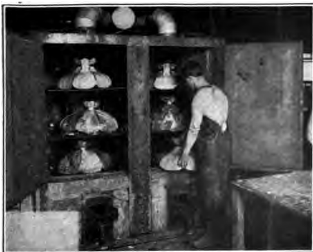
Fig. 180. Gas Fired Oven for Decorated Lamp Shades
