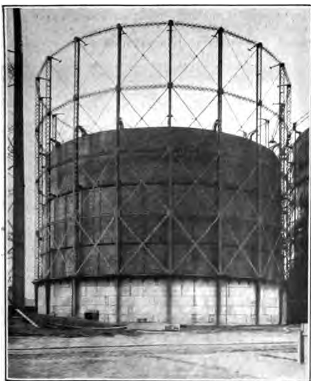
Fig. 117. Multiple-Lift Type of Holder
