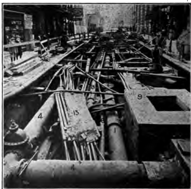
Fig. 324. A Difficult Problem in Main Laying
