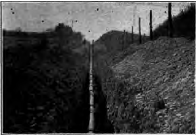
Fig. 156. Typical Trench Dug with a Modern Machine
