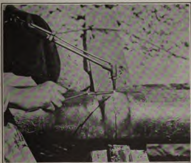
Fig. 350. Welding Steel Main with Oxy-Acetylene Torch
