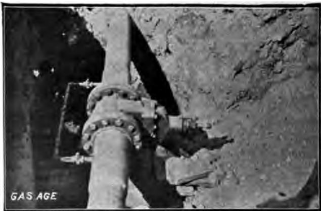
Fig. 373. By-pass and Welded Sleeve
