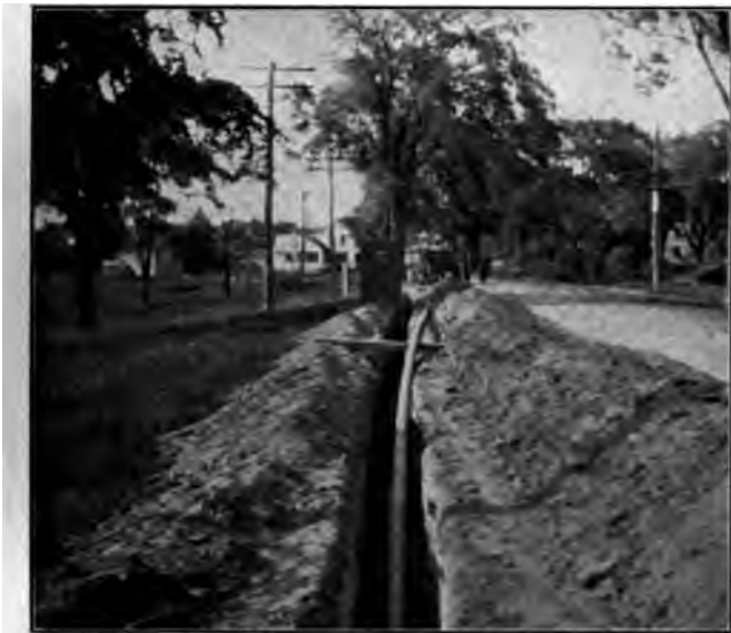
Fig. 376. Rolling Long Pipe into the Trench
