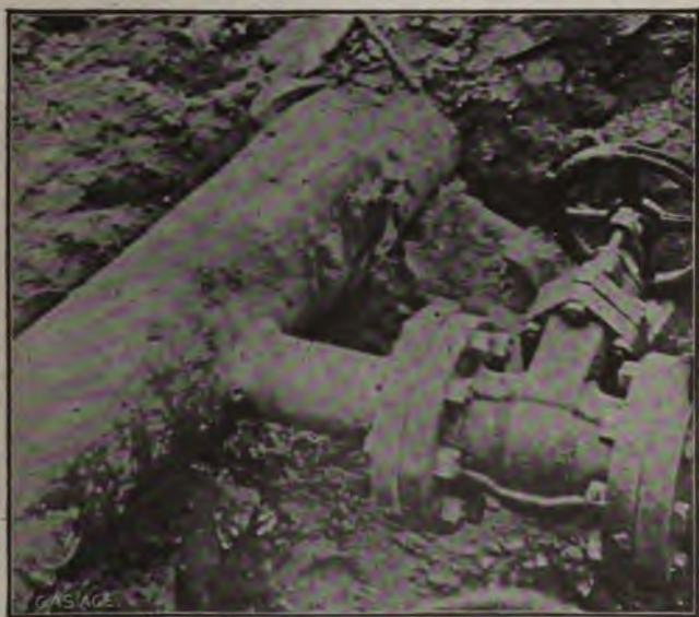
Fig. 374. A Welded Branch on High Pressure Main
