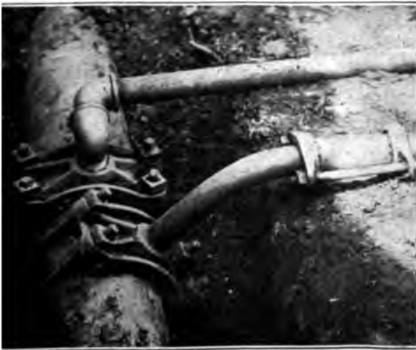
Fig. 338. Ways of Installing Service Saddles
