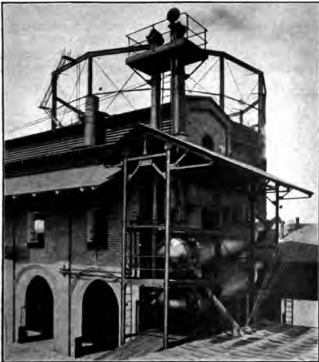
Fig. 111. Steam Boilers Fired by Waste Heat
