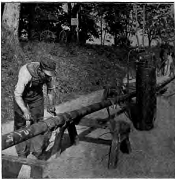
Fig. 359. Clamp for Holding Pipe Ends
