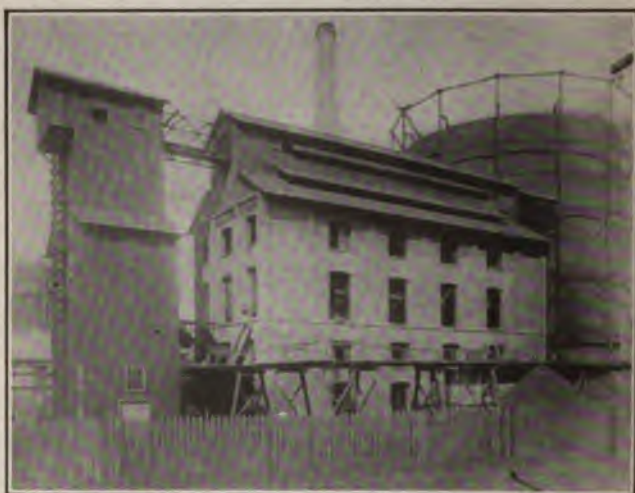
Fig. 69. Vertical Retort House at Brockton
