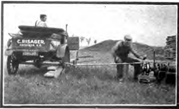
Fig. 40. Now Gasoline Power Threads the Pipe
