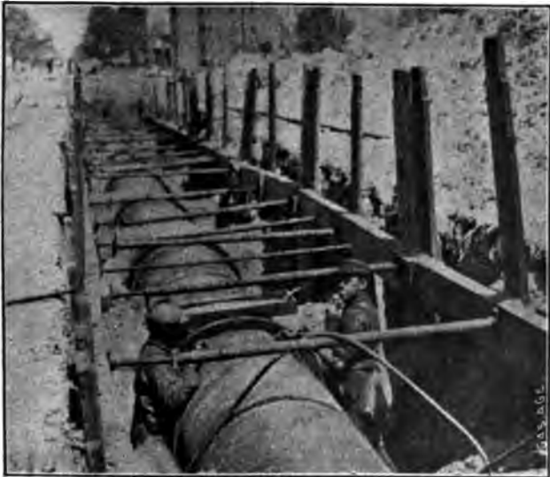
Fig. 163. Compressed Air Calking Saves Time and Labor
