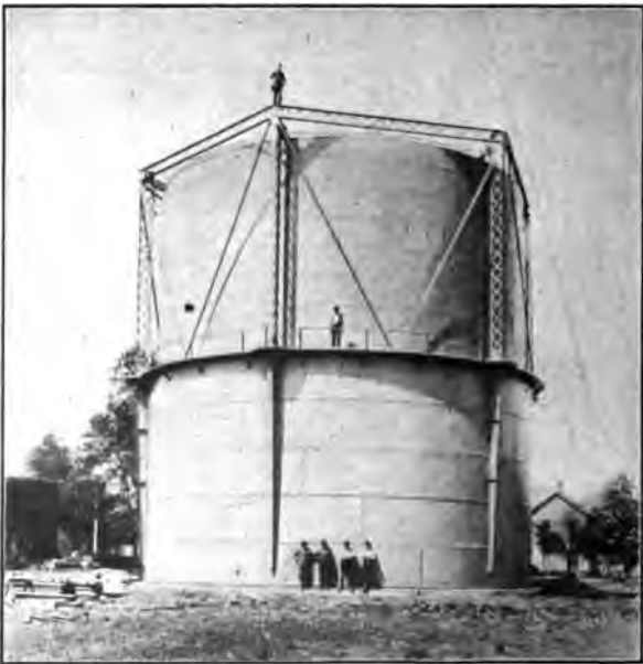
Fig. 116. Single-Lift Gas Holder in Steel Tank
