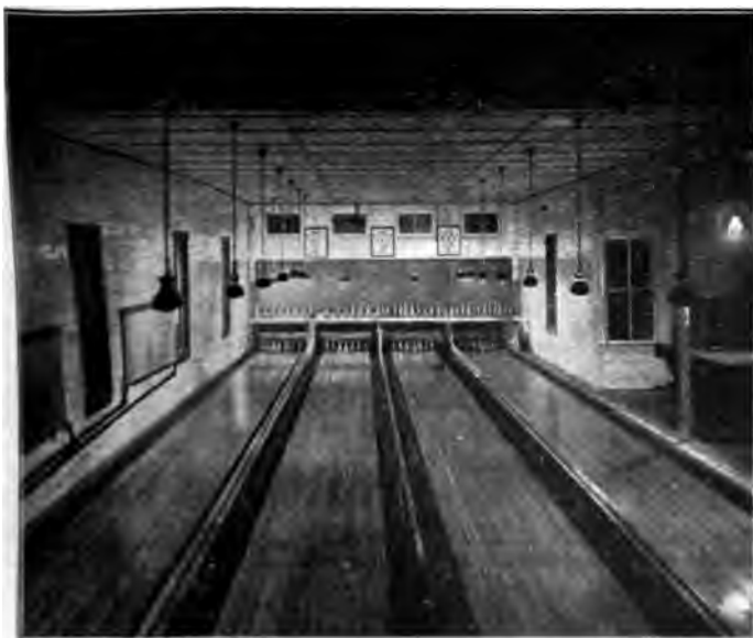
Fig. 269. Angle Reflectors, Used Also for Signs
