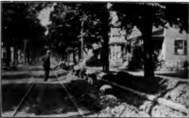
Fig. 35. The Pick-and-Shovel Street Trenching Gang
