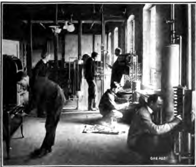
Fig. 204. Burner and Water Heater Adjustment in Baltimore
