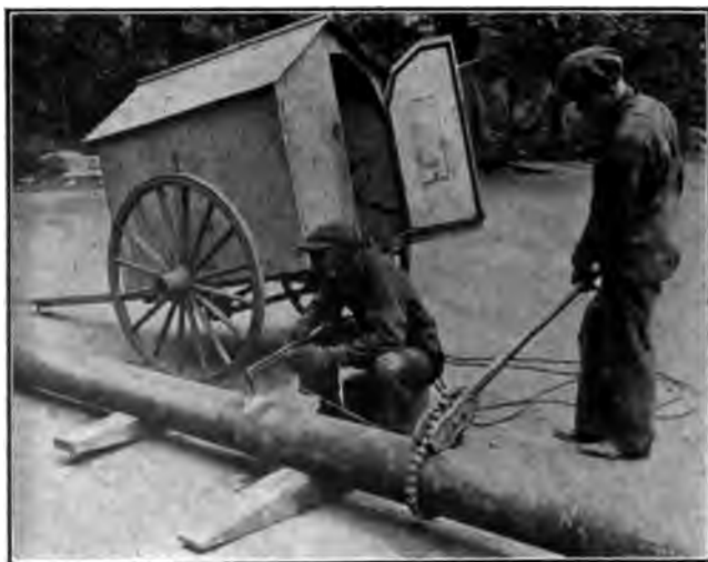
Fig. 366. Turning Pipe While Welding
