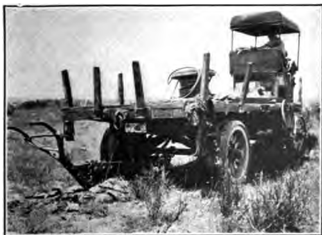
Fig. 158. Starting the Trench By Motor Truck Power
