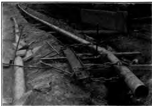
Fig. 368. Bending Welded Pipe on the Job
