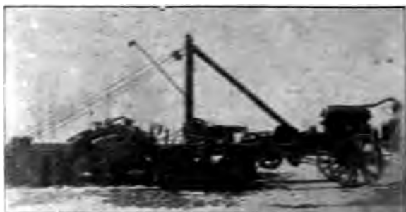
Fig. 326. An Early Form of Trenching Machine
