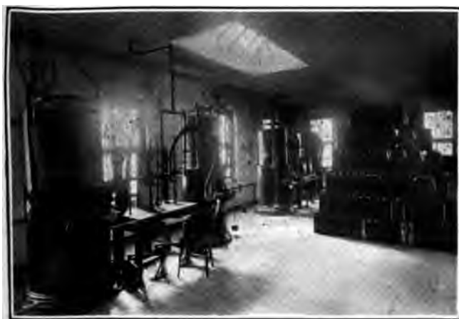
Fig. 299. A Typical Meter Testing Outfit
