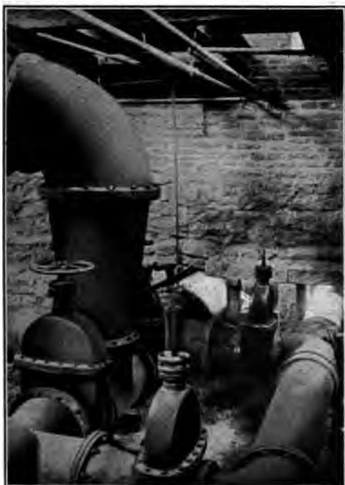
Fig. 331. A Nest of Cast Iron Pipe Specials
