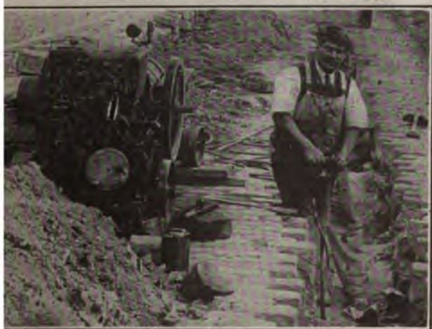
Fig. 329. Trenching by Compressed Air
