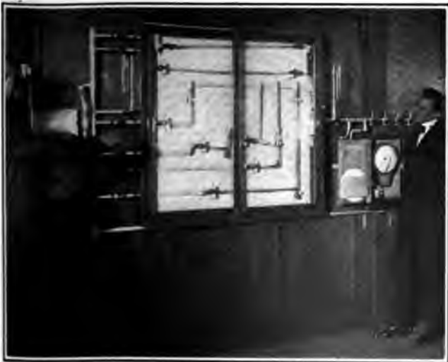
Fig. 206. House Piping Stoppage in the Baltimore School
