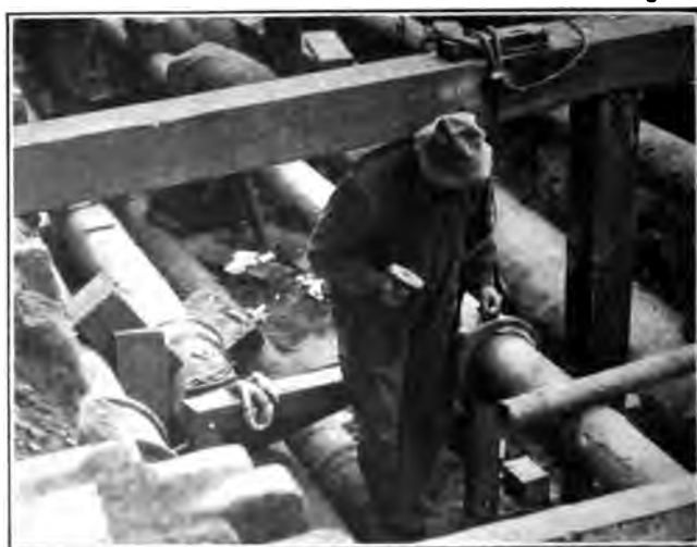
Fig. 126. Lead Caulking of City Gas Mains
