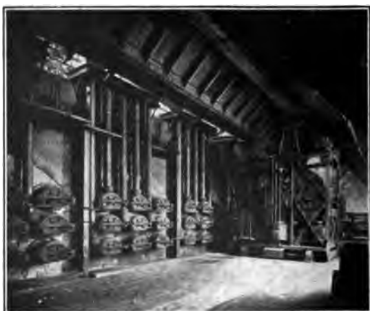
Fig. 16. Modern Mechanical Retort Charger
