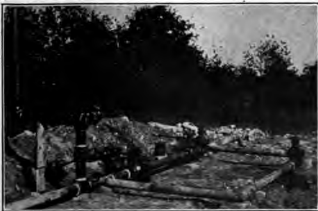
Fig. 385. Connections Made Out of 4-Inch Boiler Flues
