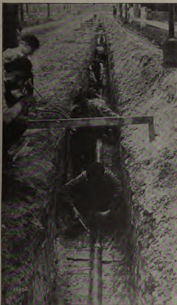
Fig. 127. Welded Joints for High Pressure Mains
