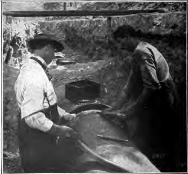
Fig. 34. Compressed Air Replaces the Hammer in Calking
