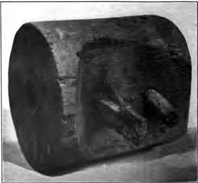
Fig. 37. The First New York Gas Main and Valve
