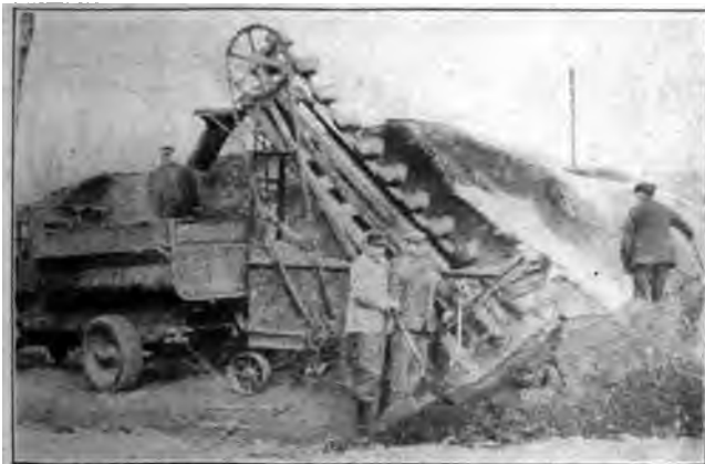
Fig. 150. Mechanical Coal and Coke Loader
