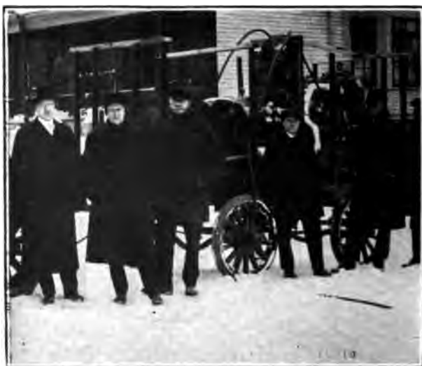
Fig. 155. A Thawing Outfit Avoids Digging Up Frozen Ground
