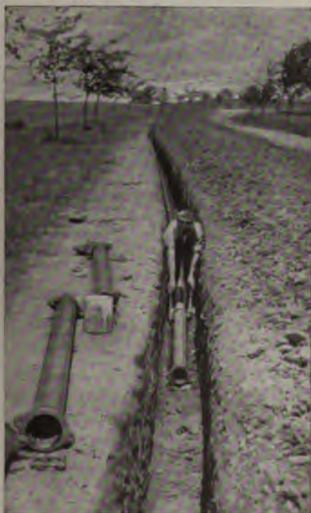
Fig. 311. Connecting Machined-Joint Cast-Iron Main
