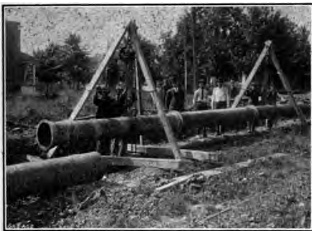
Fig. 321. Usual Method of Lowering Mains
