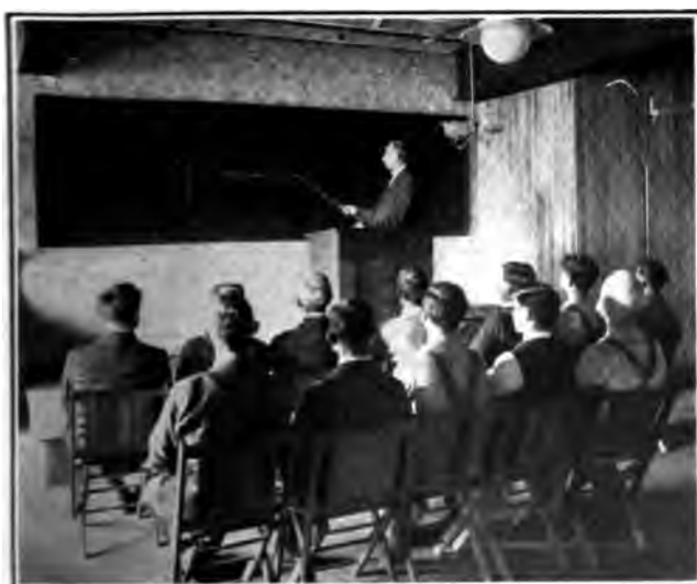
Fig. 199. Installation Instruction School at Baltimore
