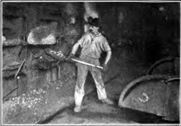
Fig. 14. Old Time Shovel Charging Retort
