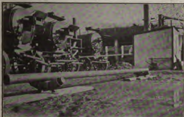
Fig. 367. Rollers for Bringing Lengths Together
