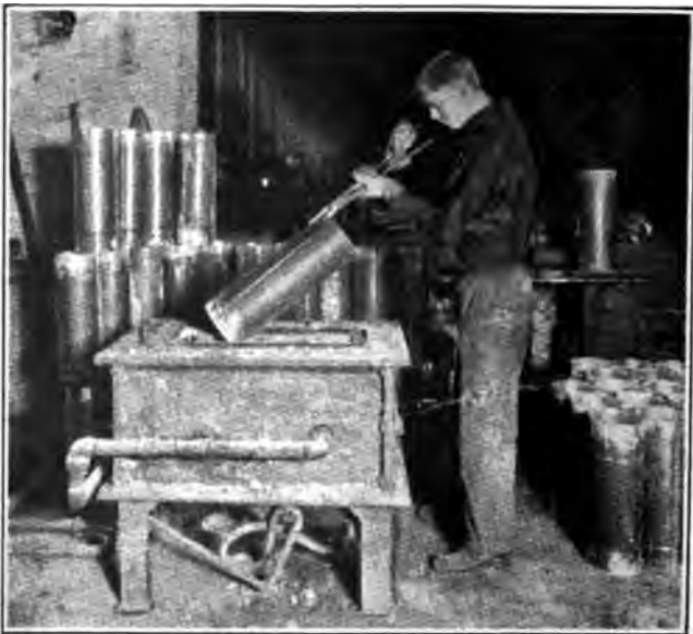
Fig. 185. Gas Heated Industrial Furnace in Operation
