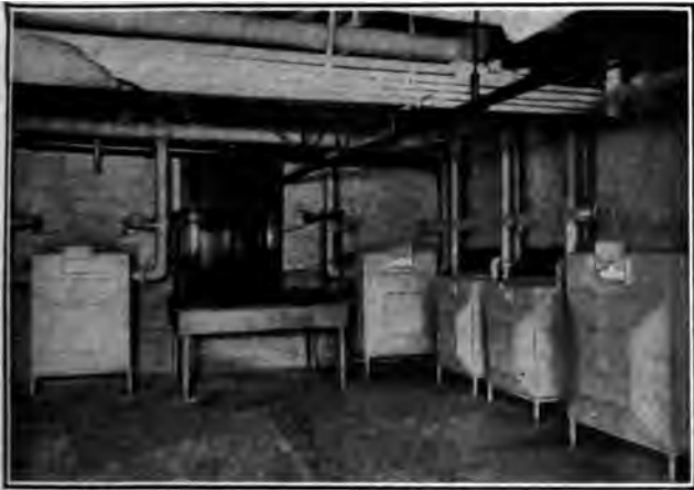
Fig. 286. Installation of Large Size Meters
