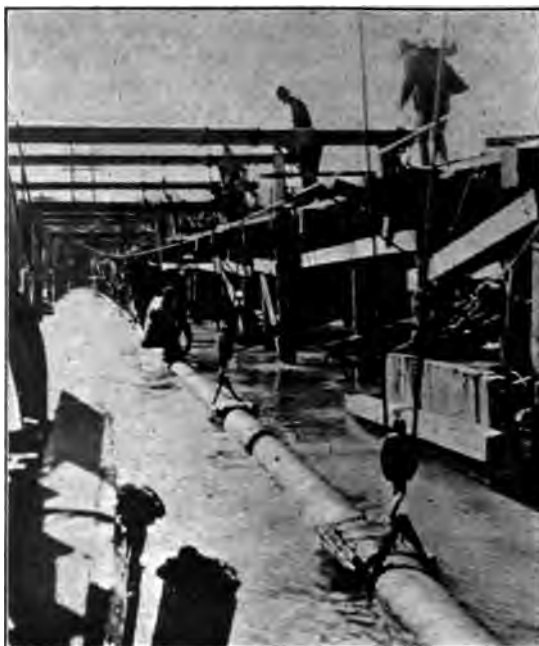
Fig. 322. Lowering Main to River-Bed Trench
