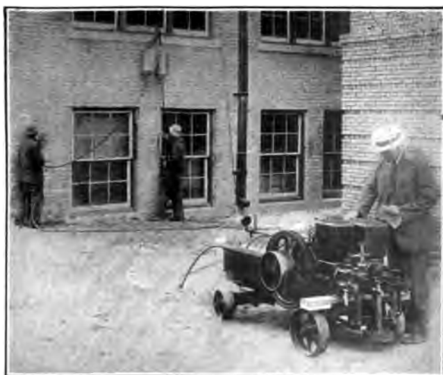
Fig. 154. Painters Save Time By Using Compressed Air
