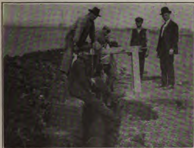
Fig. 391. Lowering the Welded Sections of Main
