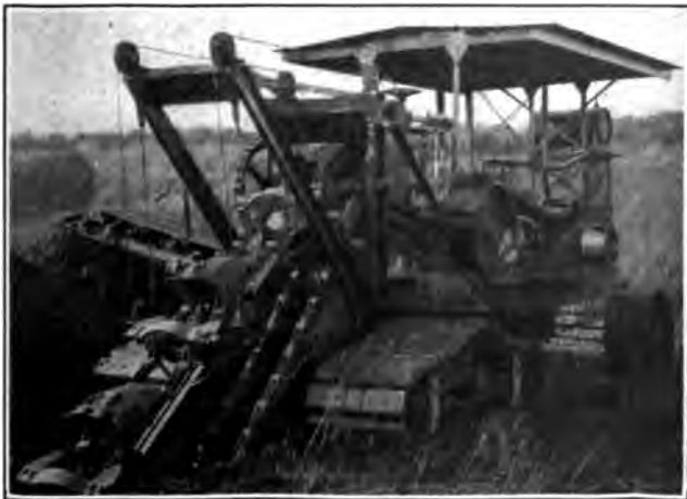
Fig. 36. Trench Excavation by Machinery
