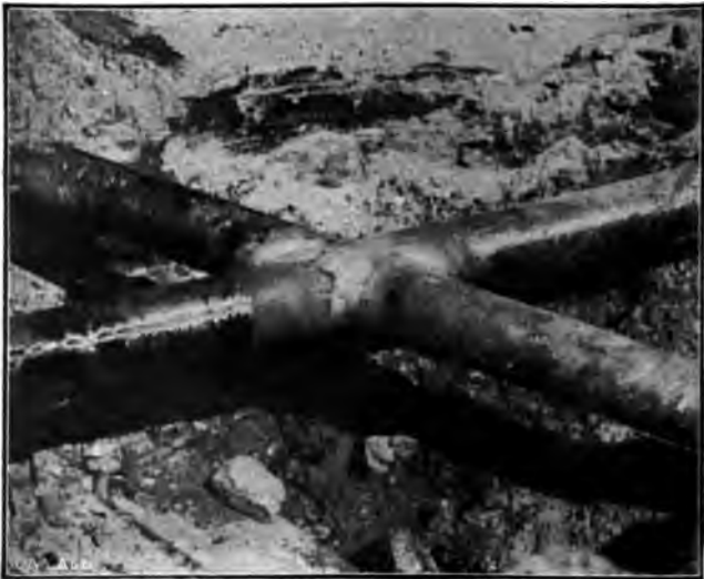
Fig. 372. A Welded Cross Made in the Field
