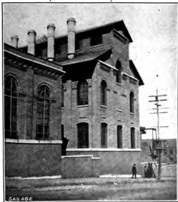
Fig. 13. Modern Gas Retort House Architecture
