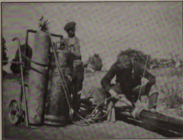
Fig. 361. Welding Equipment Used in the Field
