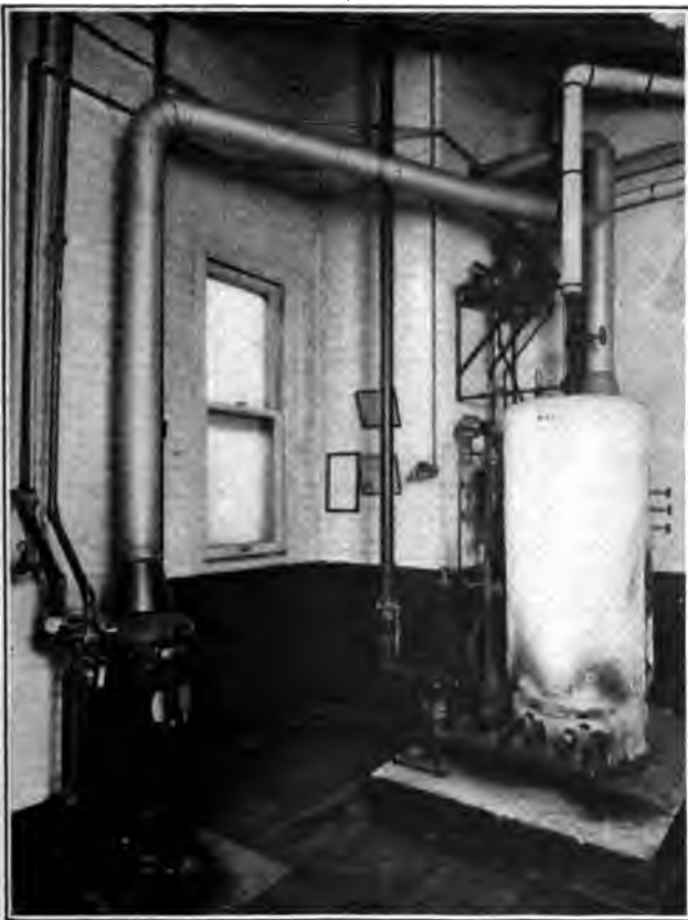
Fig. 267. Gas Heated Hot Water and Steam Supply
