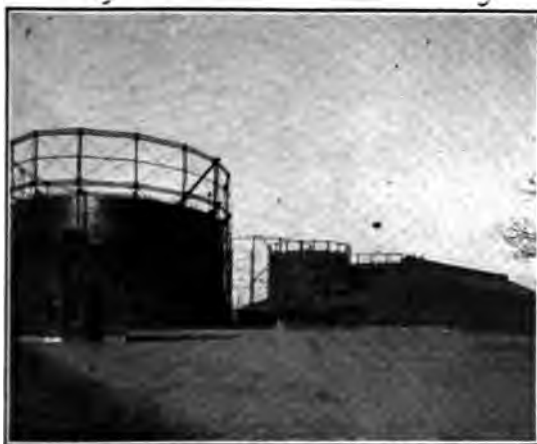
Fig. 115. Group of Gas Holders at the Works
