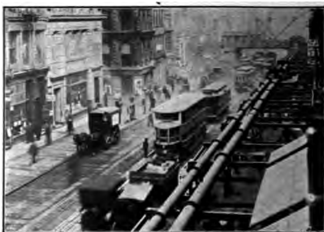
Fig. 349. A Safe Place for Gas Pipe on Busy Streets
