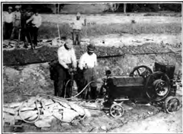
Fig. 41. Compressed Air Breaks Up Paving Over Trench
