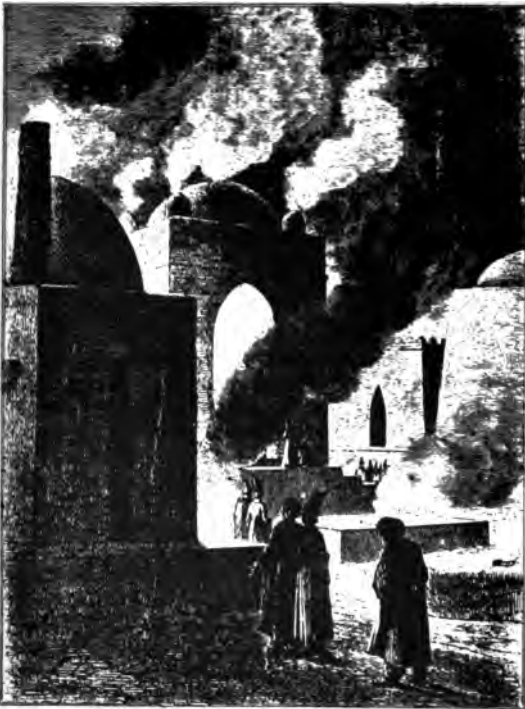
Fig. 22. Natural Gas Lighting of an Ancient Temple
