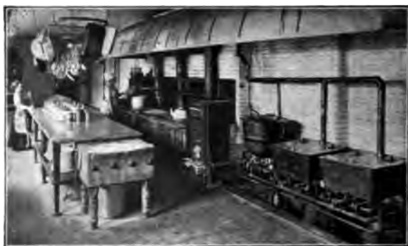
Fig. 178. Hotel Kitchen Gas Outfit With Waste Incinerator
