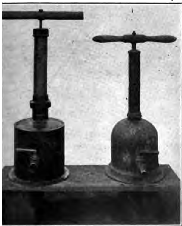
Fig. 283. Types of House Pipe Force Pumps
