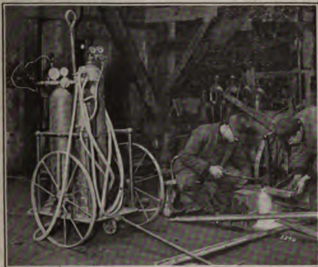
Fig. 351. Cutting Torch in Operation in Shop
