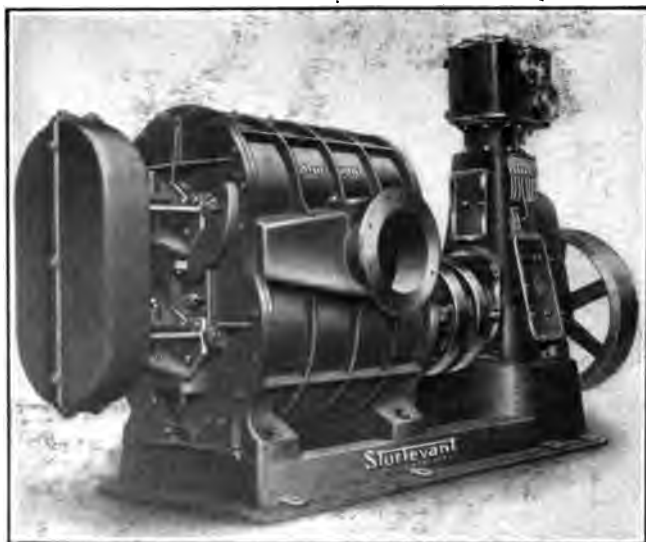
Fig. 87. A Common Form of Blower and Exhauster Drive
