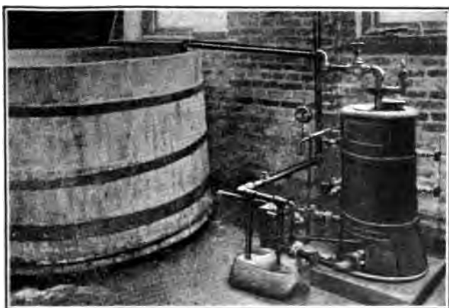
Fig. 179. Industrial Gas Fired Steam Generator
