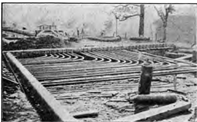
Fig. 348. Device for Muffling Pressure Pulsations
