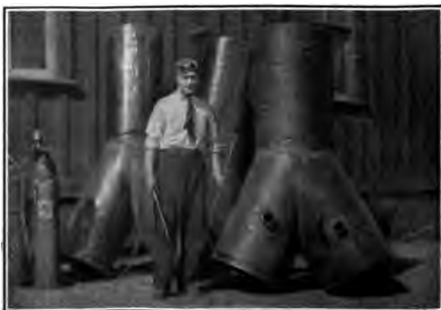
Fig. 381. Welded “Y” Branches of Large Size
