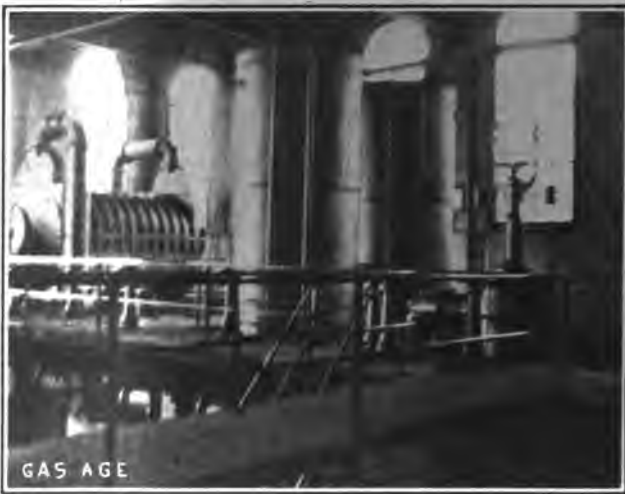
Fig. 93. Scrubber, Washer, Condenser and Tar Extractor
