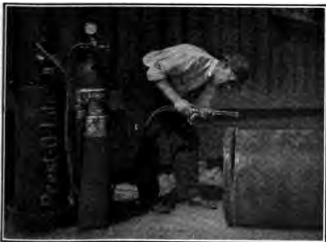
Fig. 162. Easy and Rapid Way to Cut Pipe
