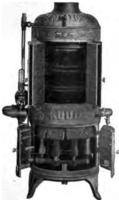
Fig. 266. Casing for Fig. 265 with Doors Open
