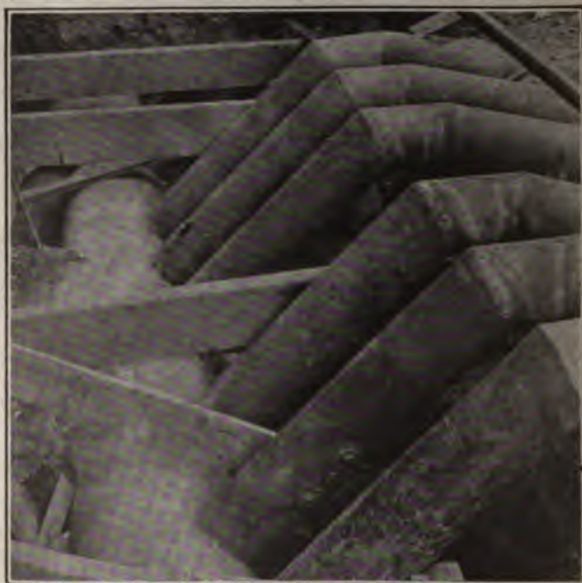
Fig. 319. Examples of Welded Main Branches
