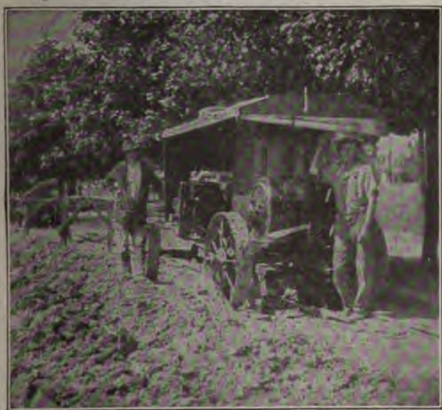
Fig. 325. Two Compressor Outfits for Main Work
