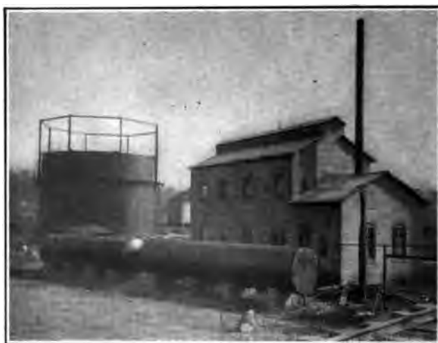
Fig. 118. Holder and High-Pressure Distribution Tanks
