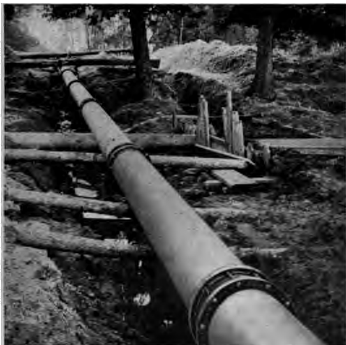
Fig. 315. Dresser Coupling for Plain-End Pipe
