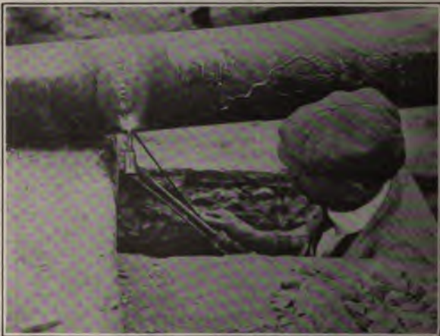
Fig. 364. Welding the Under Side of a Gas Main
