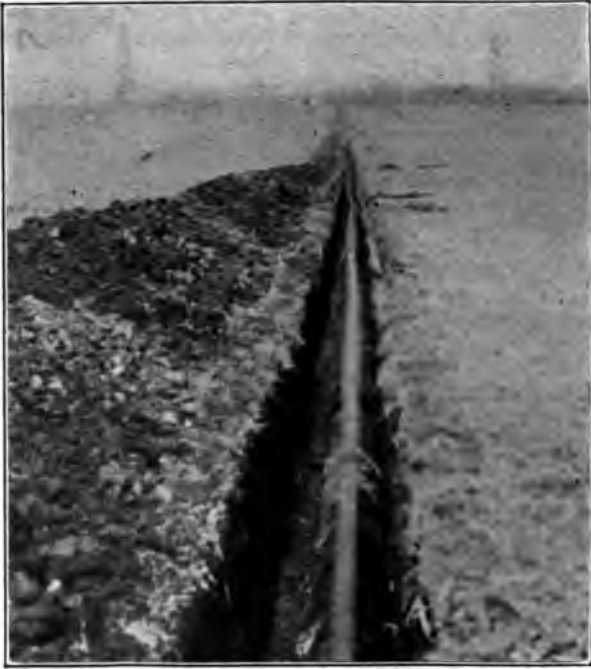
Fig. 392. Slack in Main Forced into the Trench
