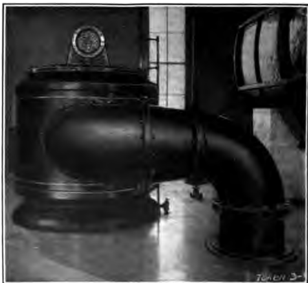
Fig. 105. Rotary Meter, Philadelphia Gas Works
