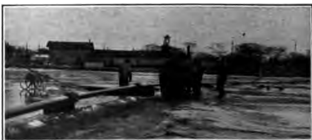
Fig. 370. Welding Main Before Lowering Through Ice
