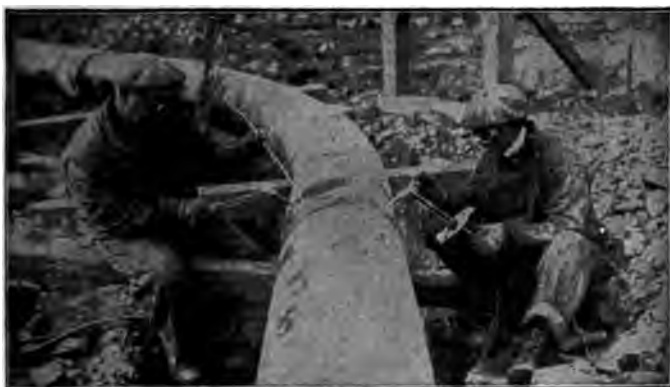
Fig. 365. Expediting the Welding of a Joint
