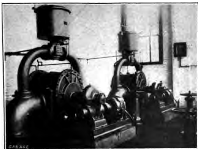
Fig. 79. Exhausters Drawing Gas from Retorts
