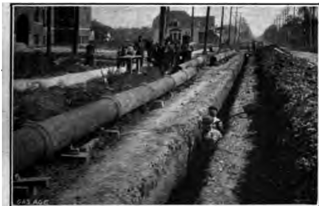
Fig. 309. Laying Cast-Iron Mains
