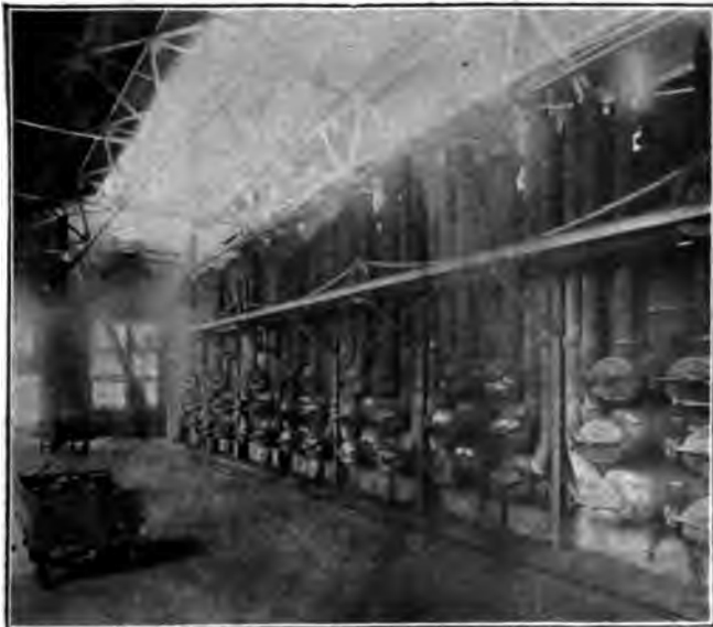
Fig. 66. Front of Coal Gas Retort Benches
