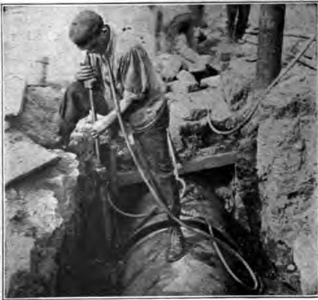
Fig. 161. Tamping with Compressed Air Saves Work
