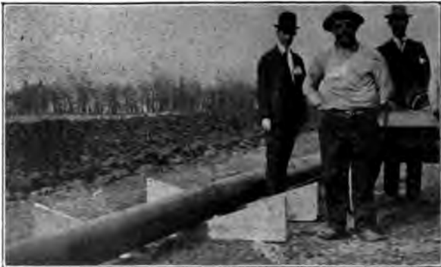
Fig. 390. Wedges for Lining Up Pipe to Make Joint
