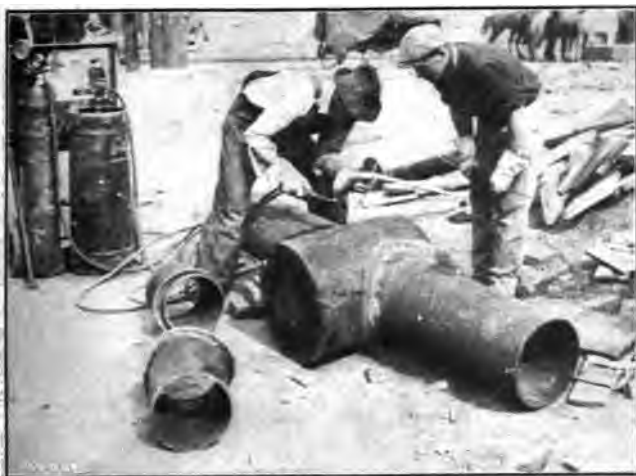
Fig. 136. Drip of Ordinary Design Welded on the Job
