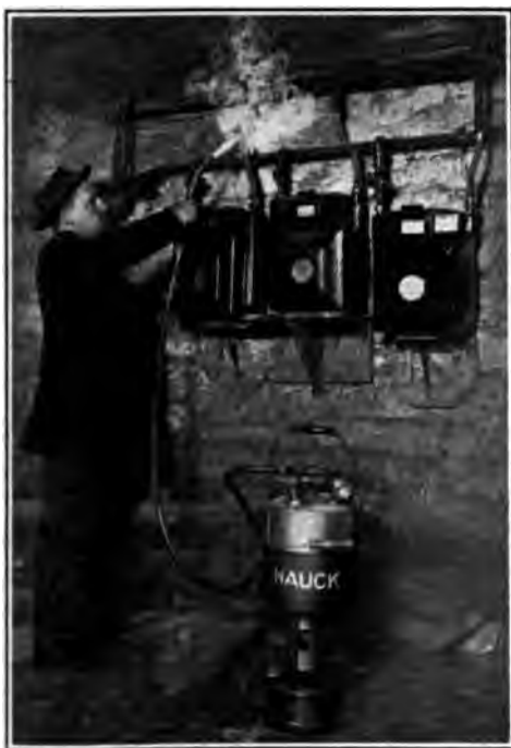
Fig. 142. Portable Steam Outfit for Pipe Thawing
