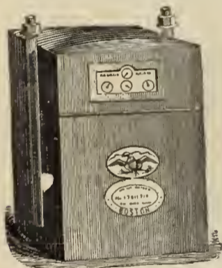
Dry Gas Meter.
