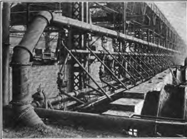
FIG. 175.—Application of powdered coal with the secondary air to the burner, using the Holbeck system.
