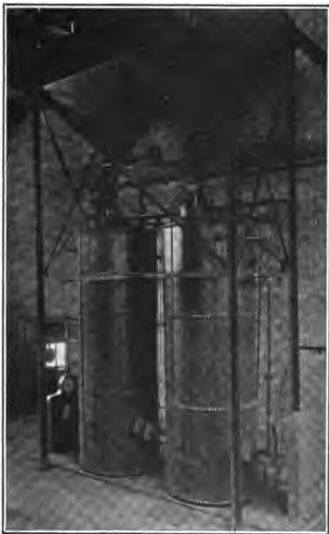
FIG. 136.—Pair of blowing tanks, mounted on platform scales, for Quigley air-transport system.
