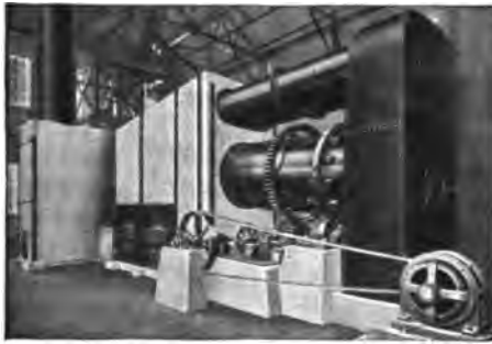
FIG. 164.—Fuller-Lehigh indirect fired dryer.
