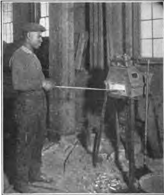
FIG. 362.—Surface combustion rivet heater; width of opening, 5.5 inches; output 100 pounds per hour.
