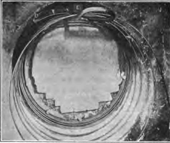
FIG. 364. —Furnace interior of installation shown in Fig. 363.
