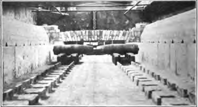
FIG. 358.—Incomplete interior of installation shown in Fig. 357.
