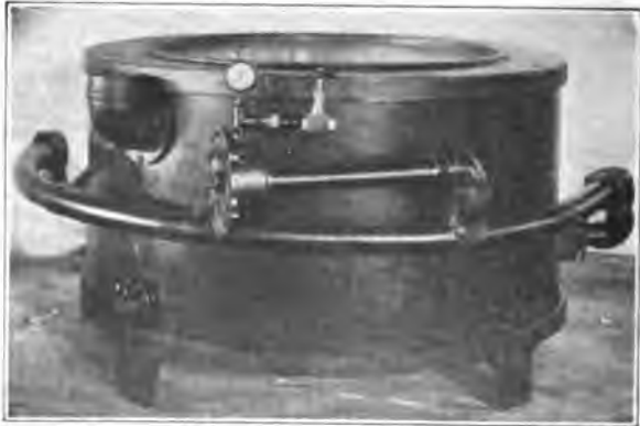
FIG. 345.—Furnace with high-pressure automatic proportioner.
