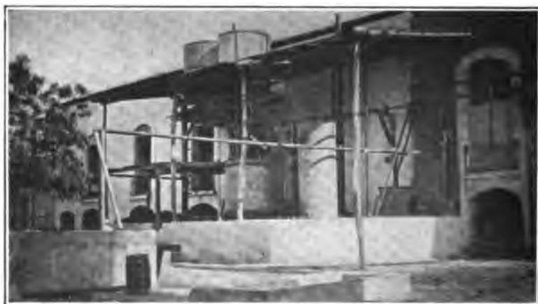
FIG. 289.—One 150-hp. type "B," fuel, wood, coconut shells, etc., at Hda Timul, Yucatan, Mexico.
