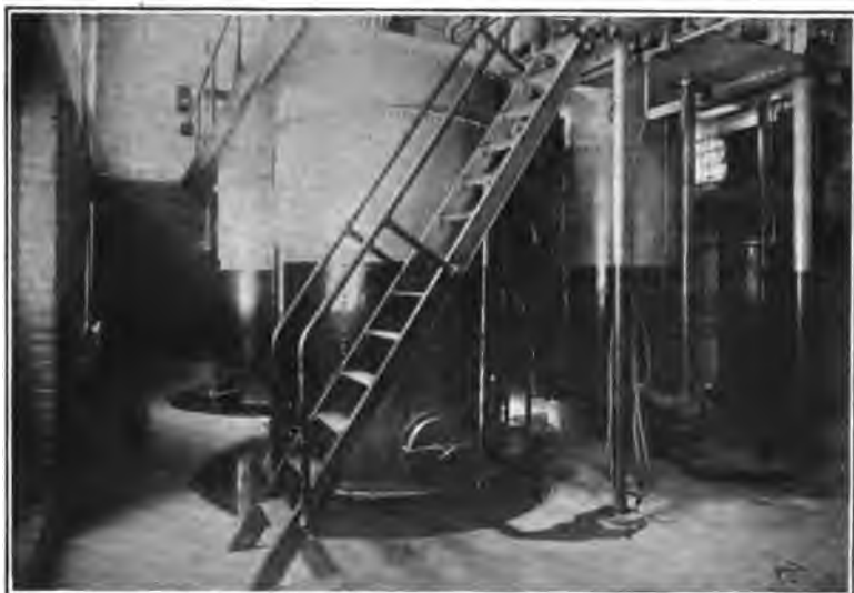
FIG. 288.—Two 100-hp. anthracite producers, Simonds Canada Saw Company, Montreal, P. Q.
