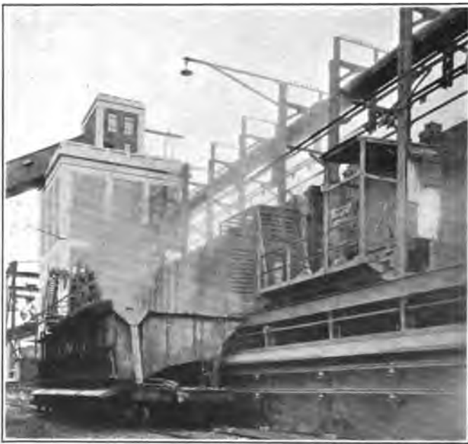
FIG. 41.—Door extractor, coke-guide and quenching-car.
