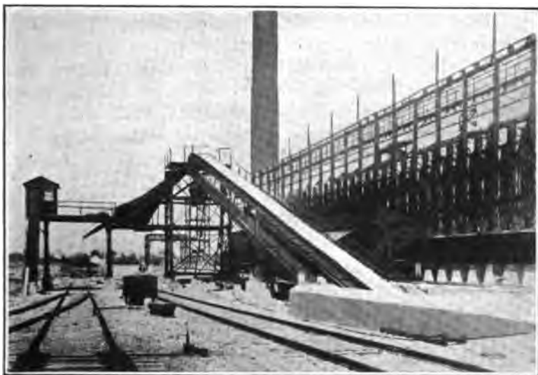
FIG. 22.—Semet-Solvay plant built for Sloss-Sheffield Steel & Iron Company, North Birmingham, Ala., showing discharge side of ovens with quenching-car and coke-belt.
