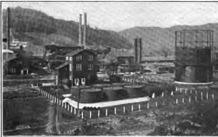
FIG. 100. —General view of by-product plant, Clinchfield Carbocoal Corporation, South Clinchfield, Va.
