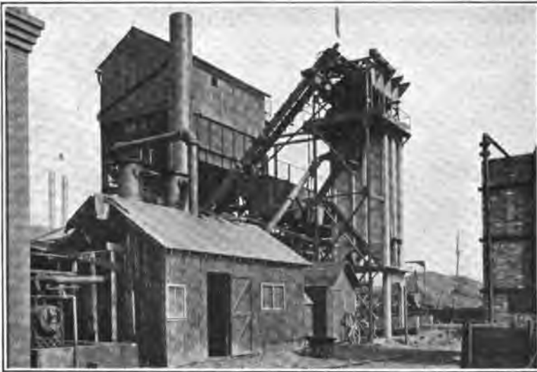
FIG. 101.—Experimental plant of the Denver Coal By-products Company.
