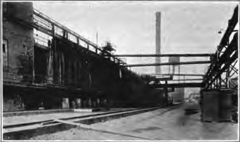
FIG. 20.—Semet-Solvay plant built for Ford Motor Company, Detroit, Mich., showing pusher side of oven with pusher in position.
