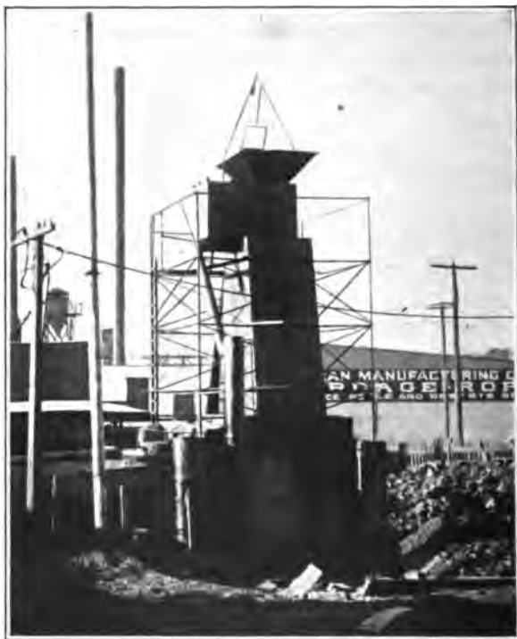
FIG. 89.—Experimental Bussey retort at Brooklyn, N. Y.
