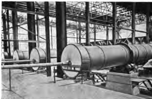
FIG. 106.—Rotary lime kilns fired with pulverized coal, Fuller-Lehigh system.
