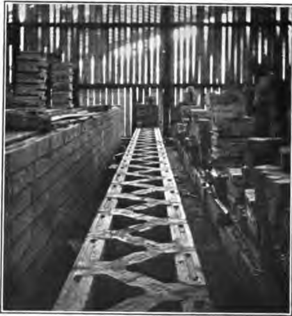
FIG. 34.—Koppers triangular flued coke-ovens under construction.
