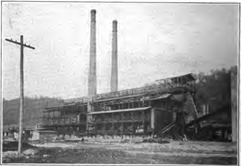
FIG. 98.—Primary retorts in the carbocoal plant of the Clinchfield Carbocoal Corporation, South Clinchfield, Va.
