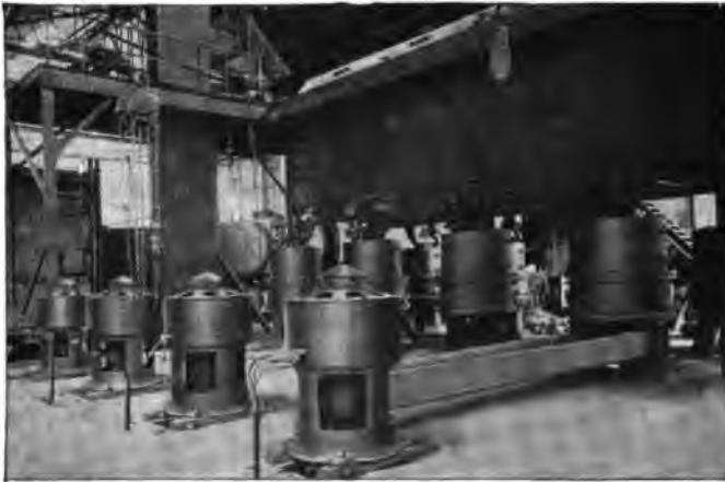
FIG. 122.—Installation of Fuller mills belted to vertical motors.
