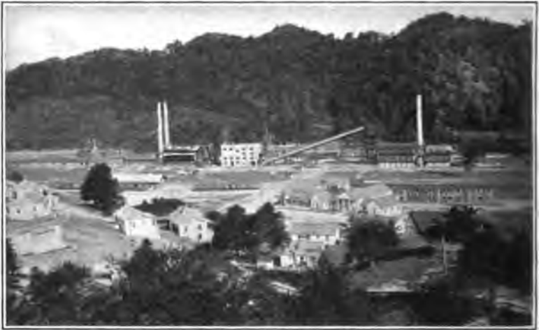
FIG. 97.—General view of the carbocoal plant of the Clinchfield Carbocoal Corporation, South Clinchfield, Va.
