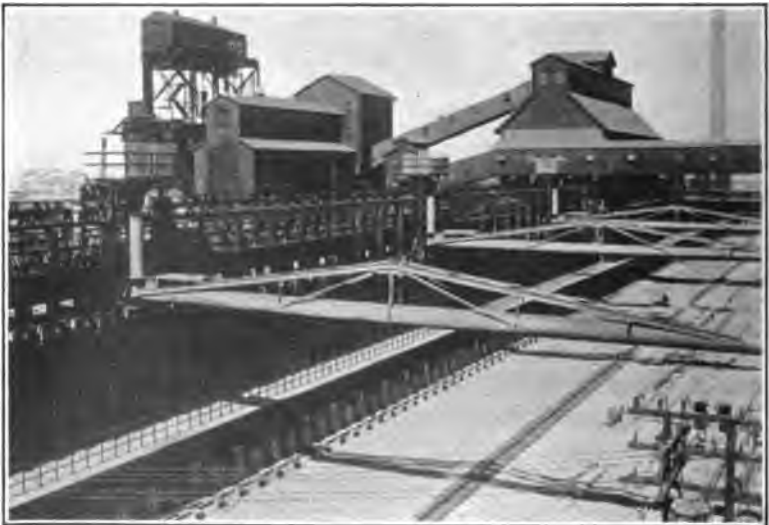
FIG. 21.—Semet-Solvay ovens built for Steel & Tube Company of America, Indiana Harbor, Ind., showing general arrangement of ovens and coal-handling equipment.
