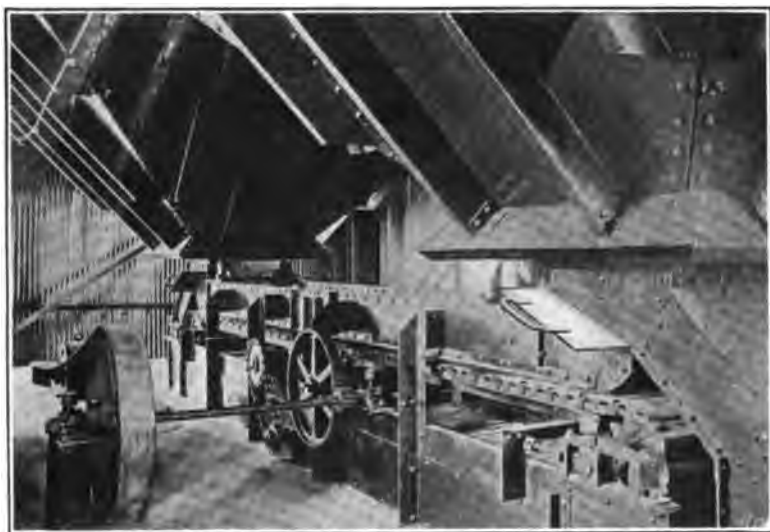
FIG. 37.—Coal-mixer for by-product coke plant.
