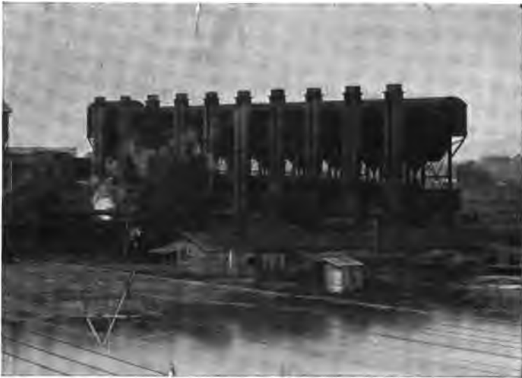
FIG. 82.—Installation of Mond by-product gas producers at Fushun Colliery. Coal bins are located above the producers.
