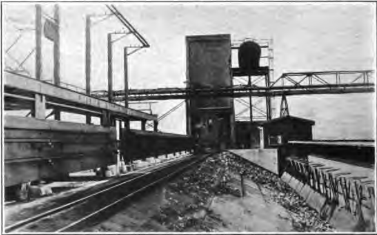
FIG. 42.—Coke-quenching station and wharf.
