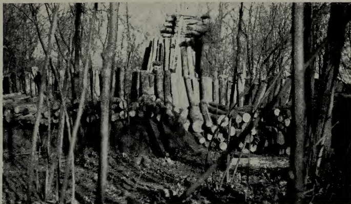
Constructing the chimney
