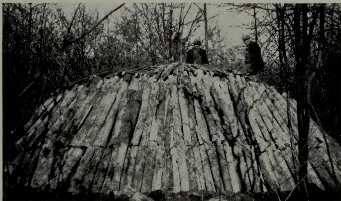
Pit ready for covering
