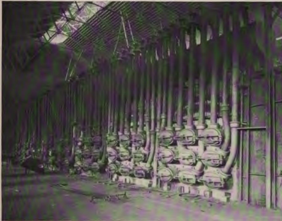
FIGURE 6. PLANT OF GAS RETORTS.
