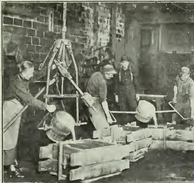
THE OLD AND THE NEW METHOD OF POURING.
