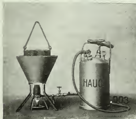
MELTING LEAD WITH HAUCK BURNER.
