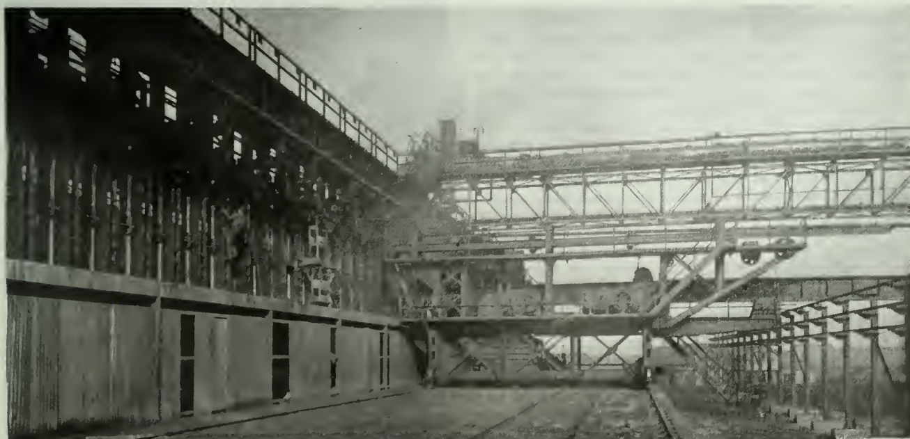
THE COKE PUSHER WHICH REMOVES THE OVEN DOORS, PUSHES THE COKE OUT ON THE OTHER SIDE INTO THE QUENCHING CAR AND THEN LEVELS DOWN THE FRESH CHARGE.
