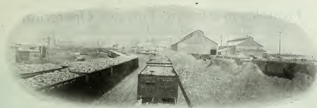
THE COAL STOCK PILES, SHOWING THE ENORMOUS TONNAGE OF COAL ALWAYS ON HAND TO SUPPLY THE COKE OVEN REQUIREMENTS.
