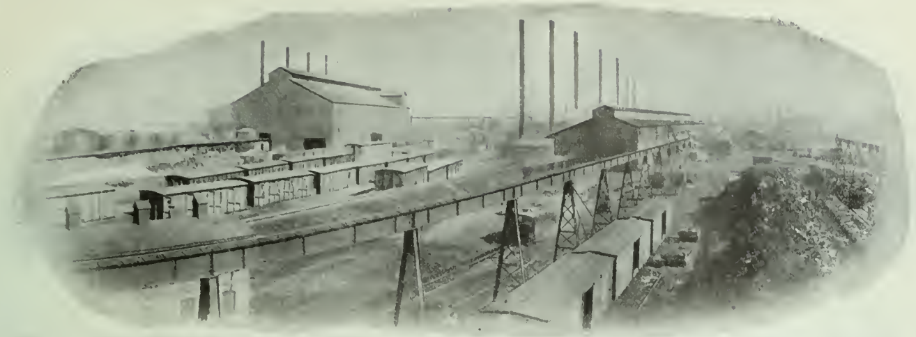
THE OPEN HEARTH STEEL FURNACES, WHICH ARE HEATED BY THE GAS AND TAR PRODUCED BY THESE MODERN OVENS. GAS AND TAR ARE TWO OF THE VALUABLE BY-PRODUCTS.
