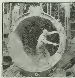
Burnt out lining showing condition of bricks after 3 heats.
