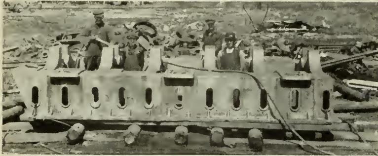
FIG. 1—SIDE VIEW OF MARINE ENGINE BED PLATE, WEIGHING 14½ TONS.
