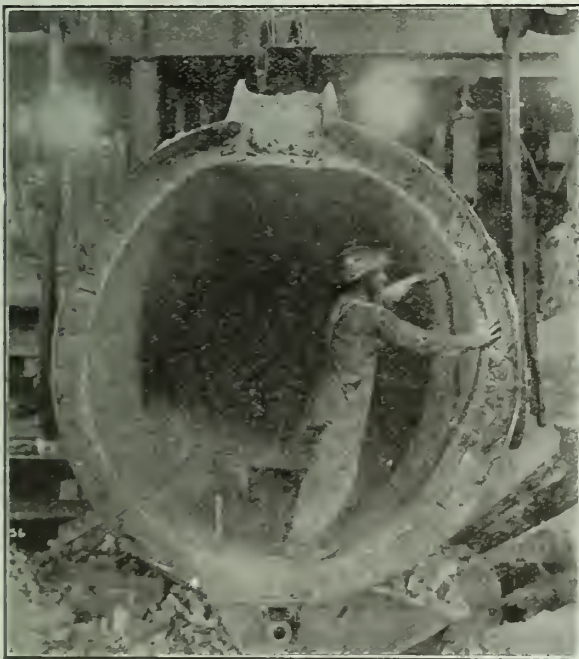
Relining a 40-ton ladle in steel foundry using Hytempite for laying up and surfacing.
