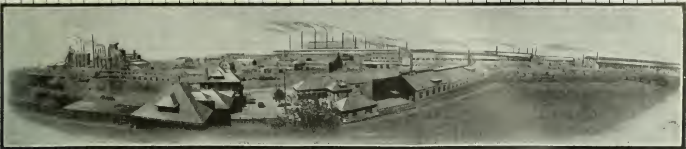
GENERAL VIEW HAMILTON WORKS HAMILTON
