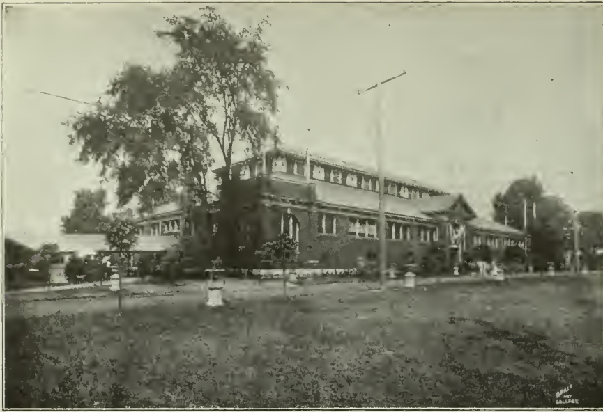
VIEW OF BUILDING NO. 1. AT LEFT IS SHOWN COVERED WALK LEADING FROM STREET CAR TO UNLOADING PLATFORM.
