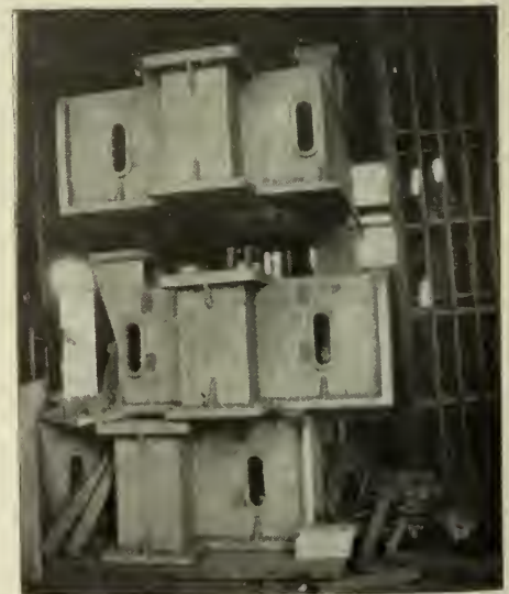
FIG. 4—THREE SECTIONS OF MARINE BED PLATE STACKED UP IN FOUNDRY. COPE ALONG SIDE USED IN PRODUCTION.
