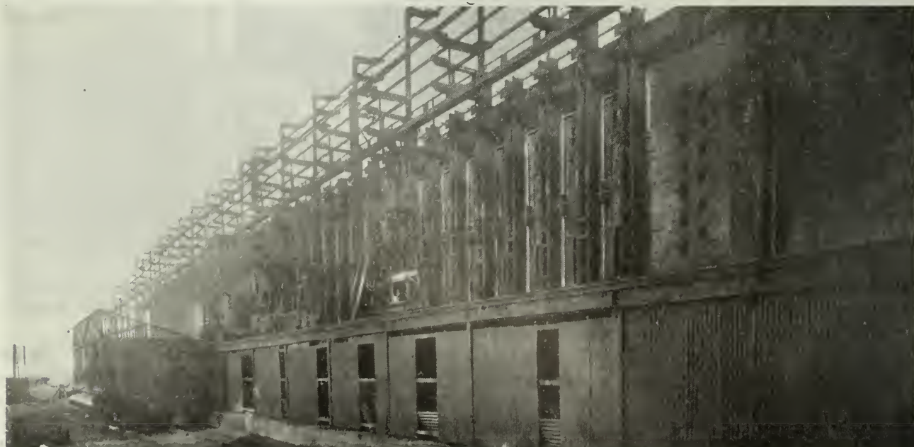
THE DISCHARGE SIDE OF THE COKE OVENS, SHOWING QUENCHING CAR.
