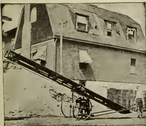
FIG. 6—ONE MAN CAN MOVE THE SCOOP CONVEYOR FROM PLACE TO PLACE.
