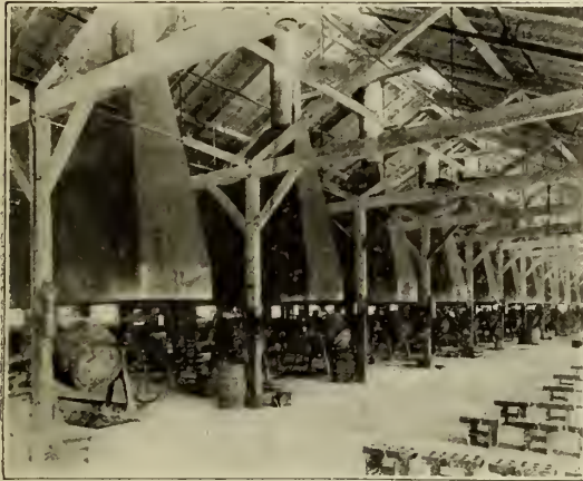
FIG. 3—PERMANENT MOLDS FOR FUSE CAPS.
