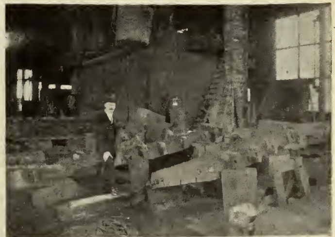
FIG. 7.—SHOWING COPES FINISHED READY FOR OVEN.
