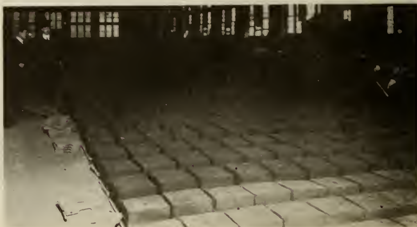
FIG. 4—MOLDER WORKING AT SNAP BENCH, ALSO FLOOR OF SNAP MOLDS.
