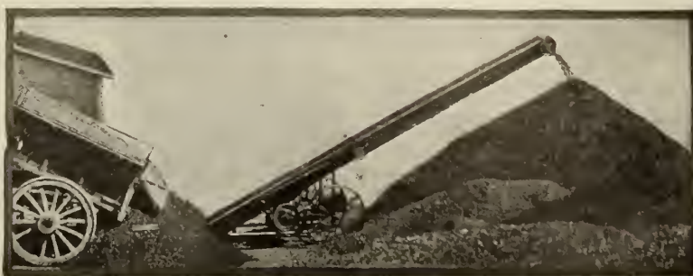
FIG. 2—UNLOADING FROM WAGON TO STORAGE PILE.
