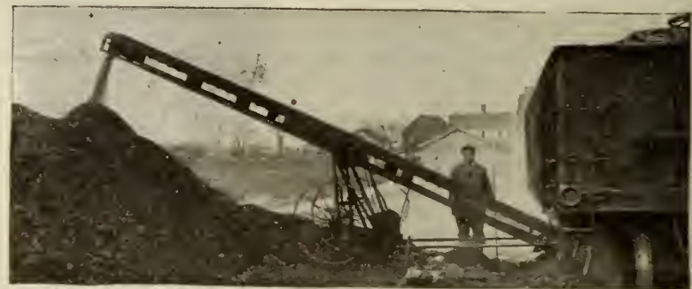
FIG. 4 UNLOADING FROM COAL CAR TO STORAGE PILE WITH A SCOOP CONVEYOR.
