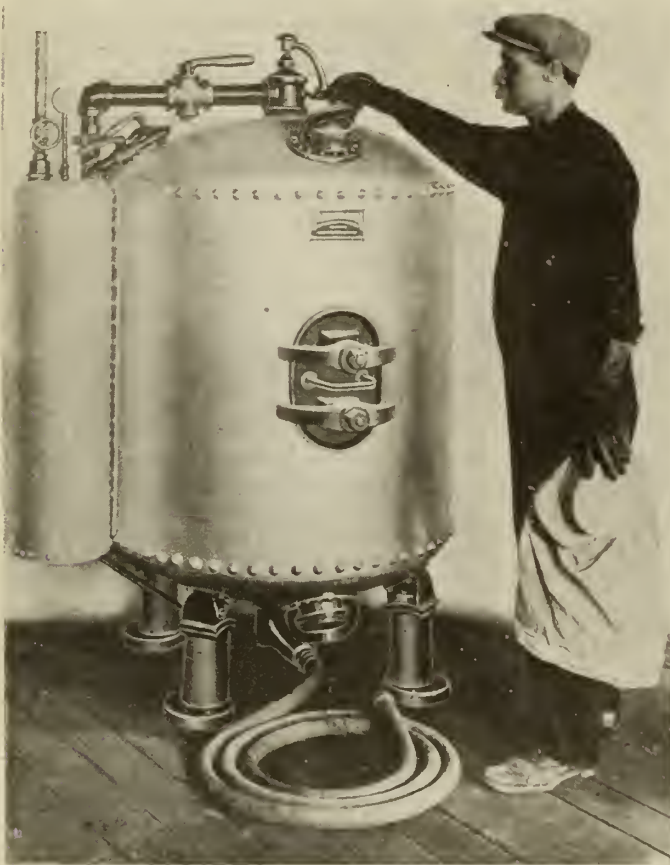
PLATE 1—HIGH PRESSURE SAND BLAST
