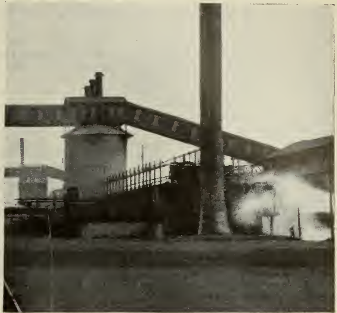
FIG. 8—ANOTHER VIEW OF THE PLANT.
