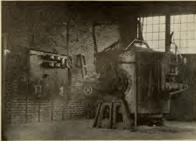
FURNACE AND CONTROL PANELS
