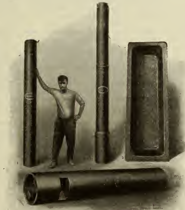
FIG. 1.—TUBES OF CAST NICHROME.
