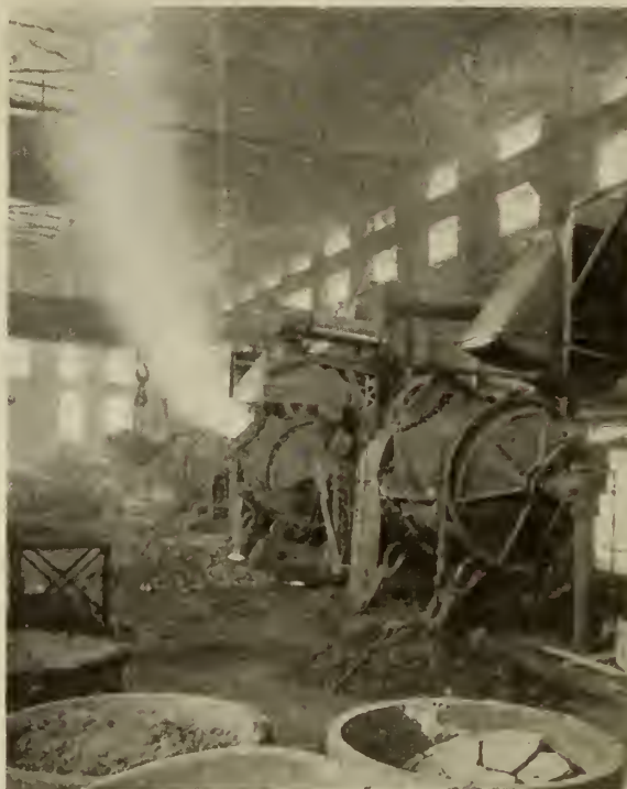
COPPER CONVERTER IN REFINERY BUILDING
