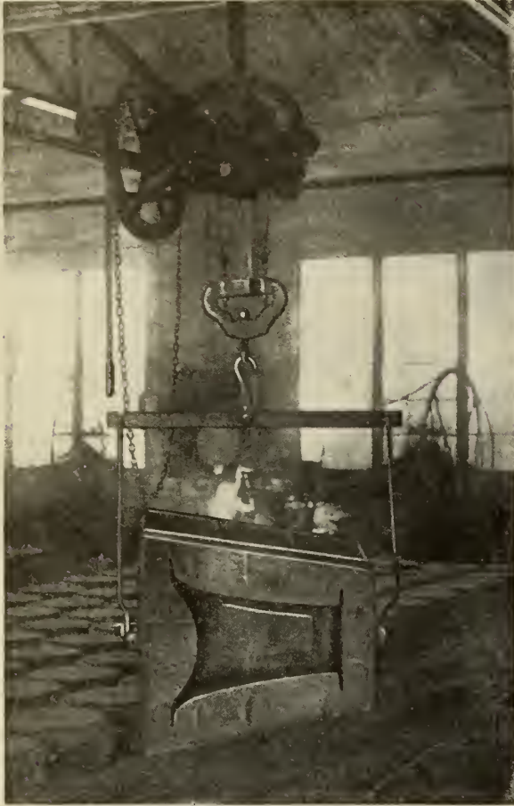
FIG. 5—POURING DEVICE USED AS A TROLLEY HOIST.
