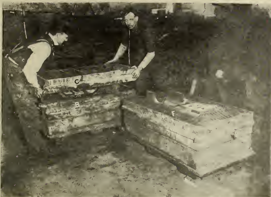
FIG. 3—SHOWING CHEEK IN POSITION AND COPE BEING LOWERED INTO PLACE.
