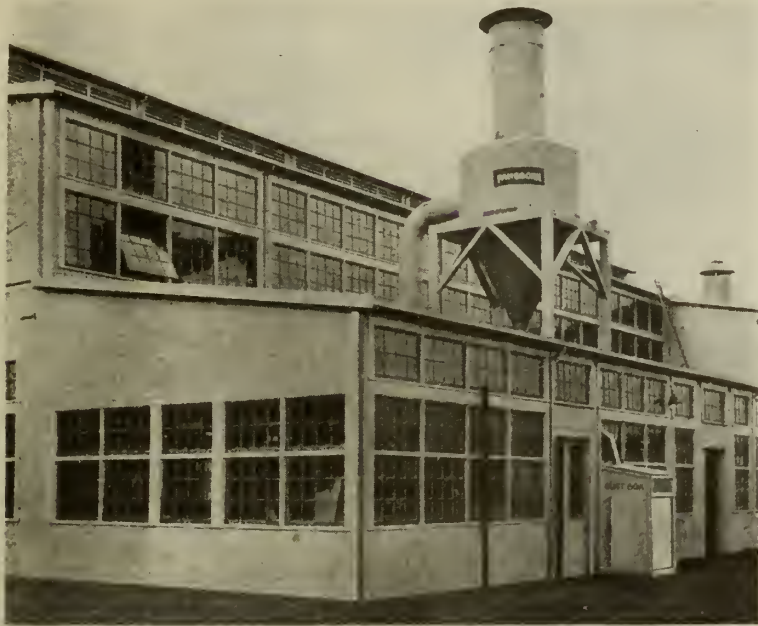
PLATE 19—CENTRIFUGAL DRY PROCESS ARRESTER
