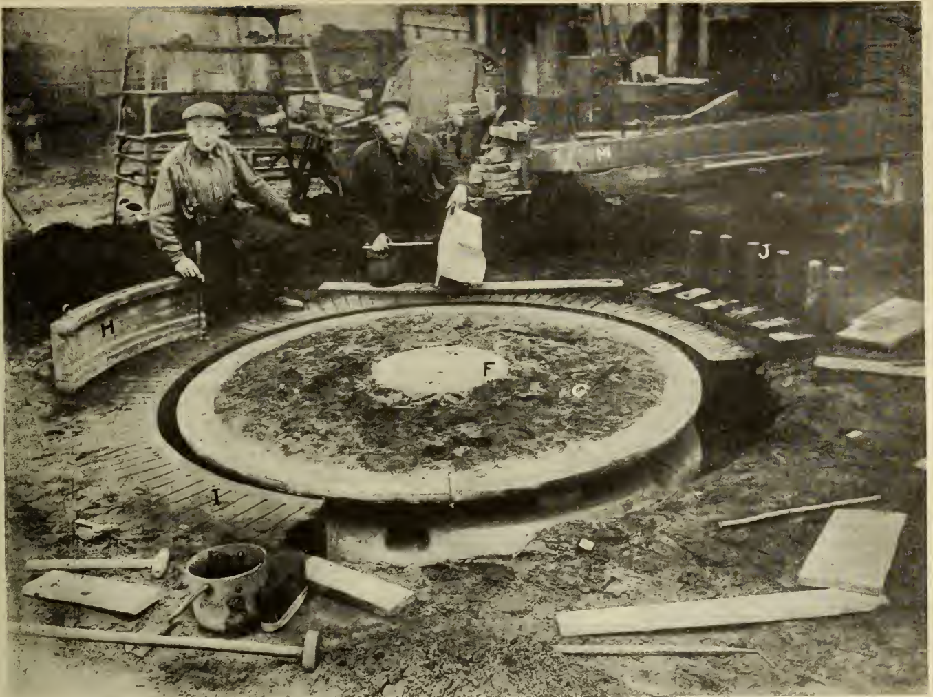
FIG. 2—SHOWING CORES REDDED IN AND RIM PARTLY RAMMED UP.
