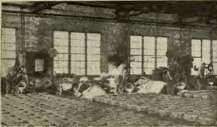
FIG. 3—POURING MOLDS BY MEANS OF OVERHEAD CRANES.
