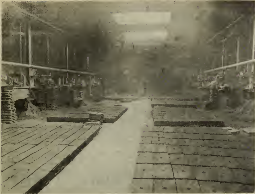
FIG. 3 SECTION OF SNAP FLOOR, SHOWING SKYLIGHTS, ALSO INDICATING THAT THE PRACTICAL MOLDER STILL HAS HIS PLACE
