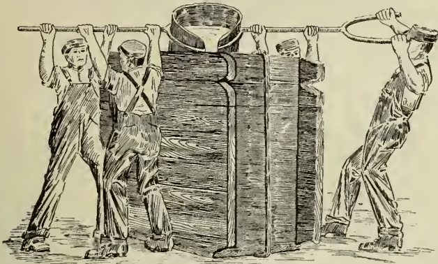
FIG. 2—SHOWING HOW HIGH MOLDS ARE USUALLY Poured.
