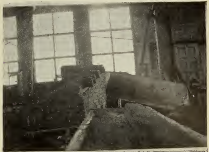
FIG. 6.—SHOWING COPE BUILT ON ONE BLADE, AND ASTERN SURFACE ON ANOTHER.
