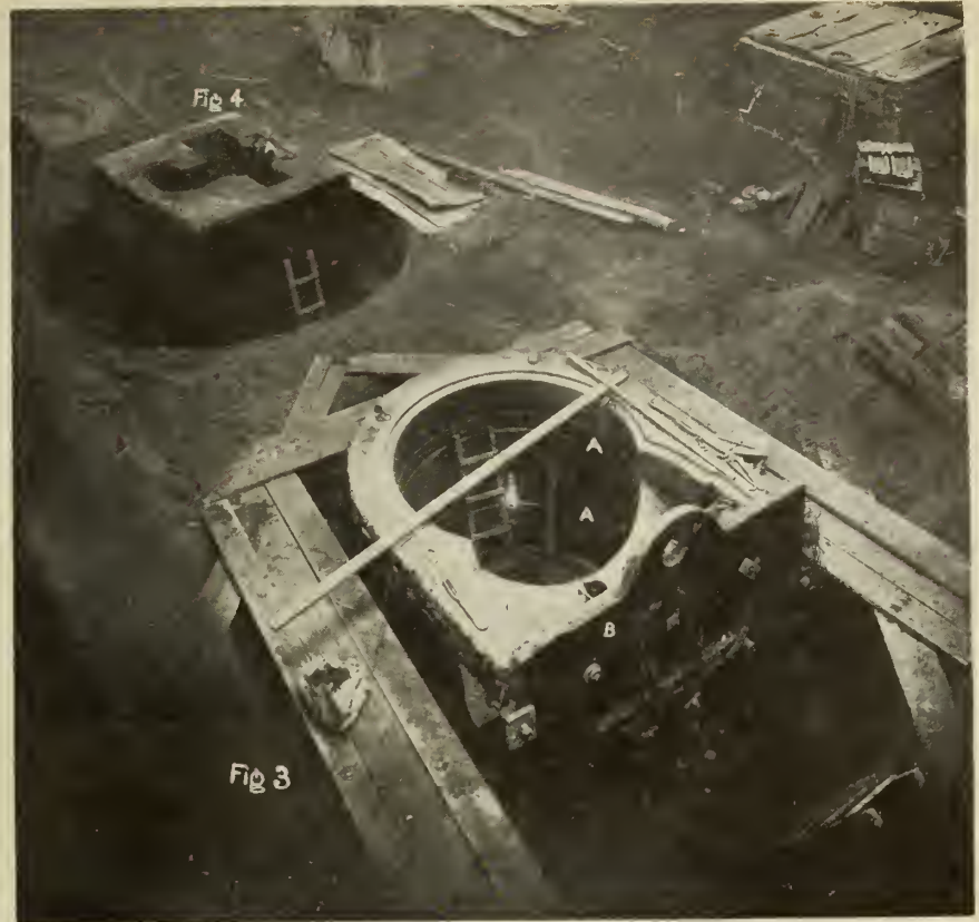
FIG. 3 IS L.P. CYLINDER MOLD WITH STEAM CHEST AND STEAM PORT CORES IN PLACE, READY TO RECEIVE MAIN CORE. FIG. 4 IS H.P. CYLINDER MOLD.
