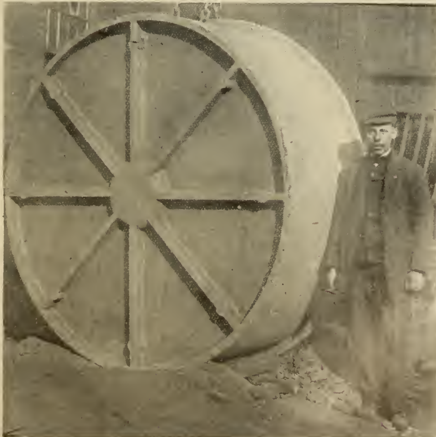
AN INTERESTING CASTING MADE IN A COMBINATION LOAM AND DRY-SAND MOLD.
