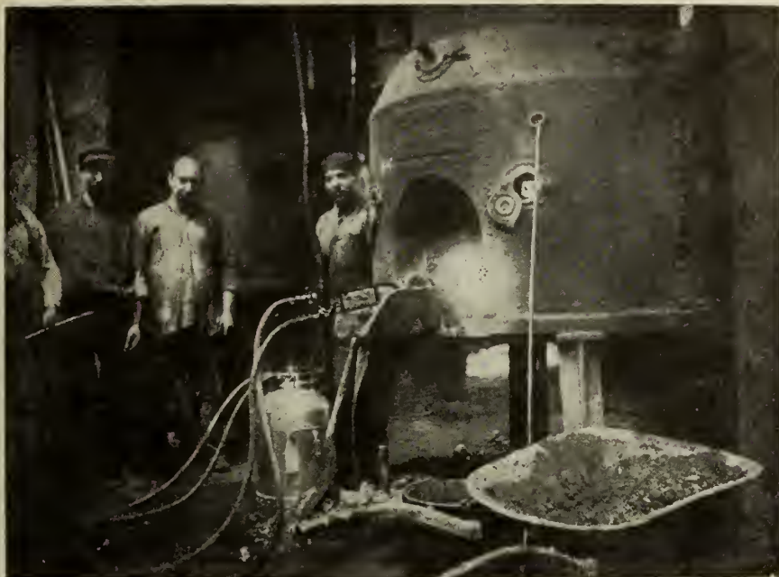
LIGHTING CUPOLA WITH PORTABLE OIL BURNER, WITHOUT THE USE OF KINDLING WOOD.
