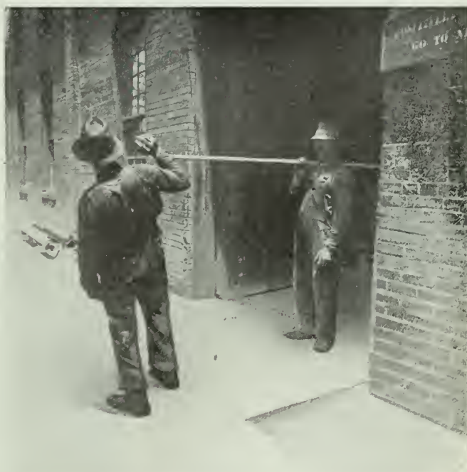
FIG. 26. SHOWING DANGER TO PASSERS BY WHEN CARRYING BARS, PIPES AND SIMILAR MATERIAL THROUGH DOORWAYS.
