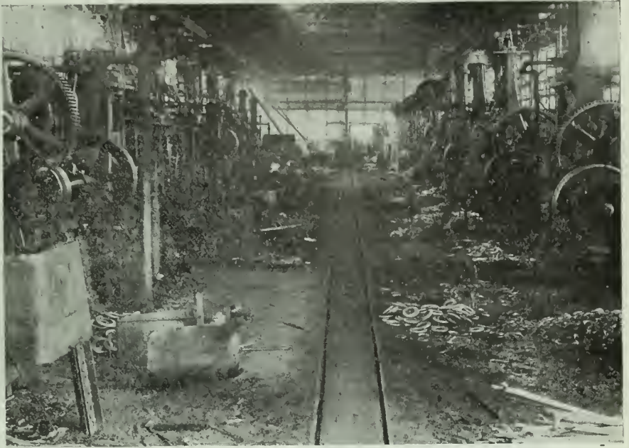
LOOKING DOWN THE CENTRE OF FORGE DEPARTMENT, PLANT NO. 2.
