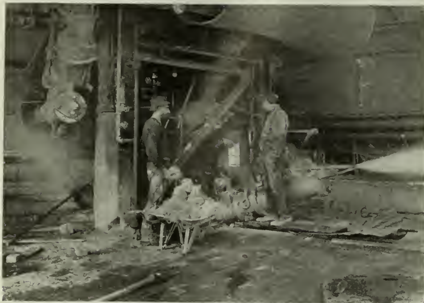
FIG. 17. UNSAFE WAY TO STOP TAPPING HOLE. Helper is using his hands and standing too near tapping hole.
