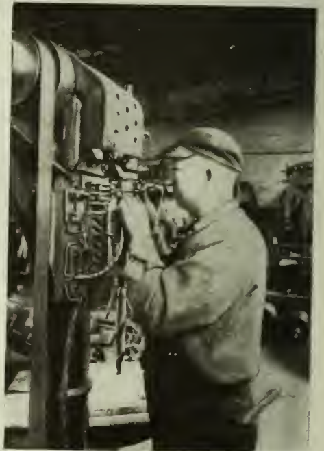
FIG. 41. ELECTRICIAN REPAIRING WIRES WITH SWITCH IN; A DANGEROUS PRACTICE.
