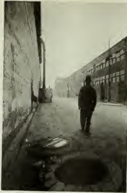
FIG. 28—WORKMAN LEAVING MANHOLE UNCOVERED
