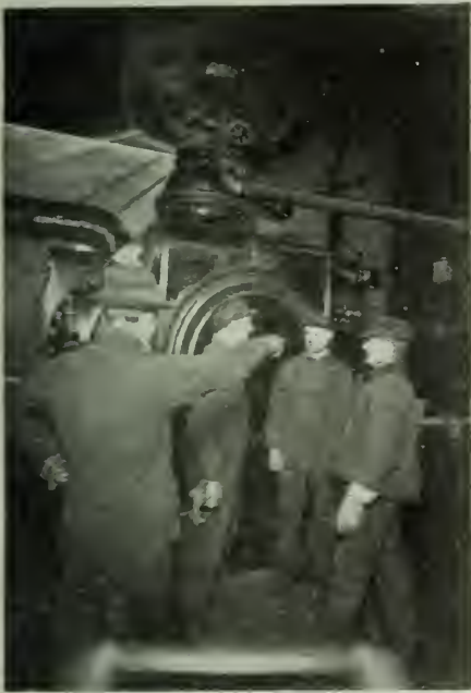
FIG. 1—FOREMAN WARNING MEN AWAY FROM CYLINDER HEAD OF STEAM ENGINE
