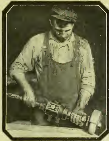
For Ramming, Grinding and Chipping Grey Iron or Steel Castings
