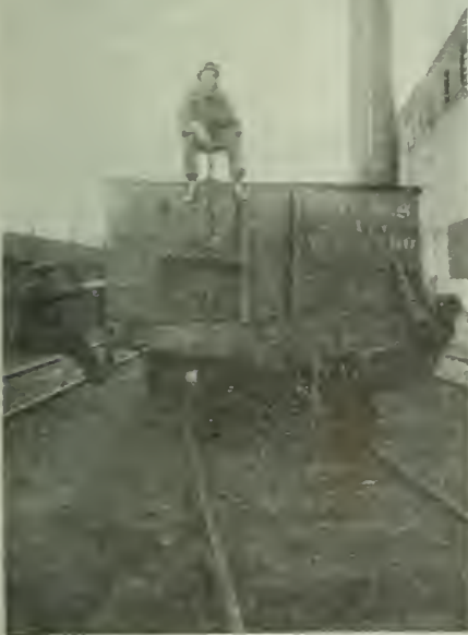
FIG. 5—UNSAFE WAYS OF RIDING ON RAILROAD CARS
