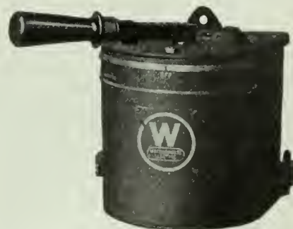
DRUM REVERSE SWITCH SUITED FOR MOUNTING DIRECTLY ON MACHINES.
