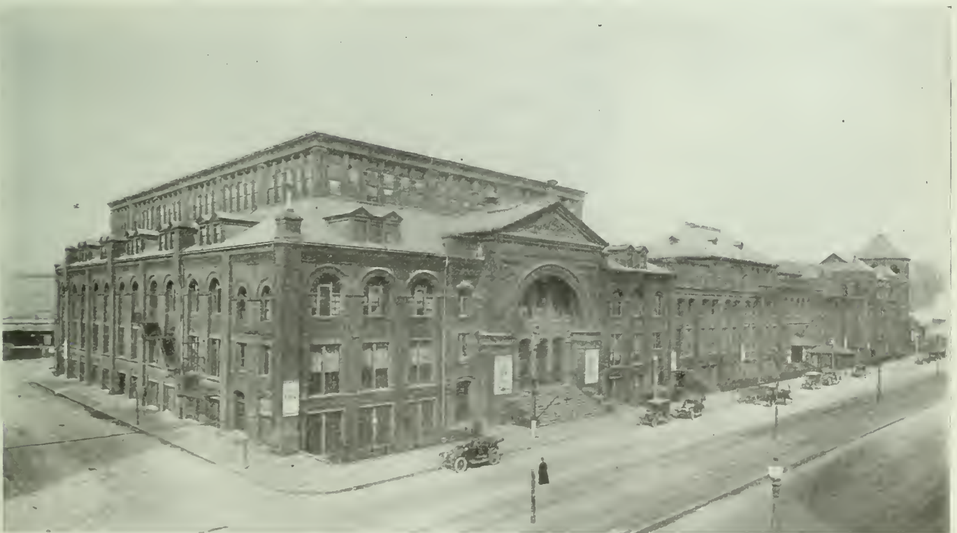
MECHANICS BUILDING, BOSTON, MASS., WHERE THE EXHIBITION OF FOUNDRY EQUIPMENT AND SUPPLIES WILL BE HOUSED.
