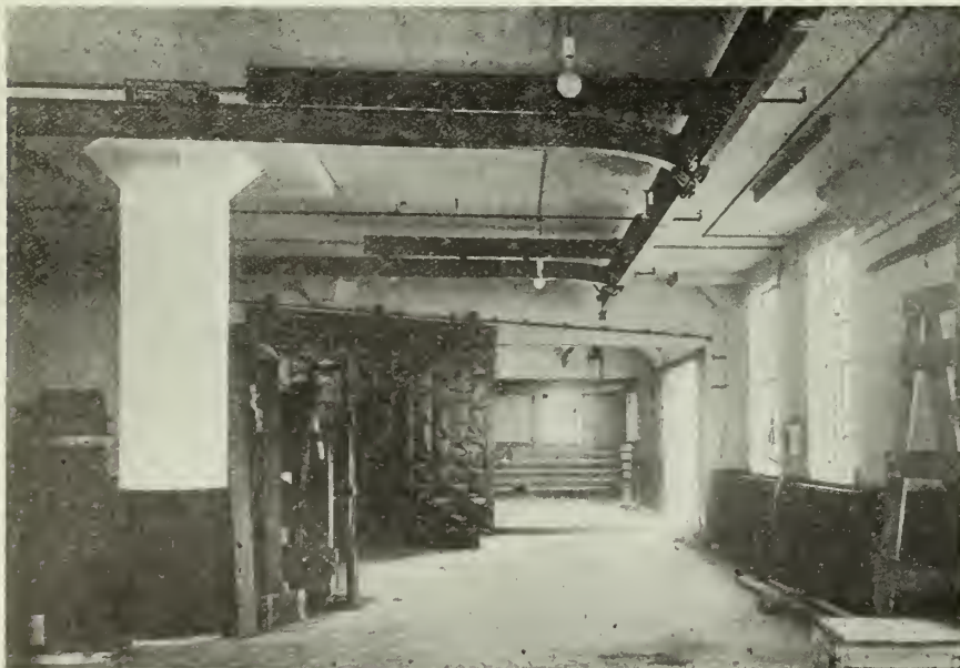
PART OF LAYOUT FLOOR IN PATTERN SHOP, SHOWING SYSTEM OF OVERHEAD RUNWAYS WITH ELEVATOR IN BACKGROUND.
