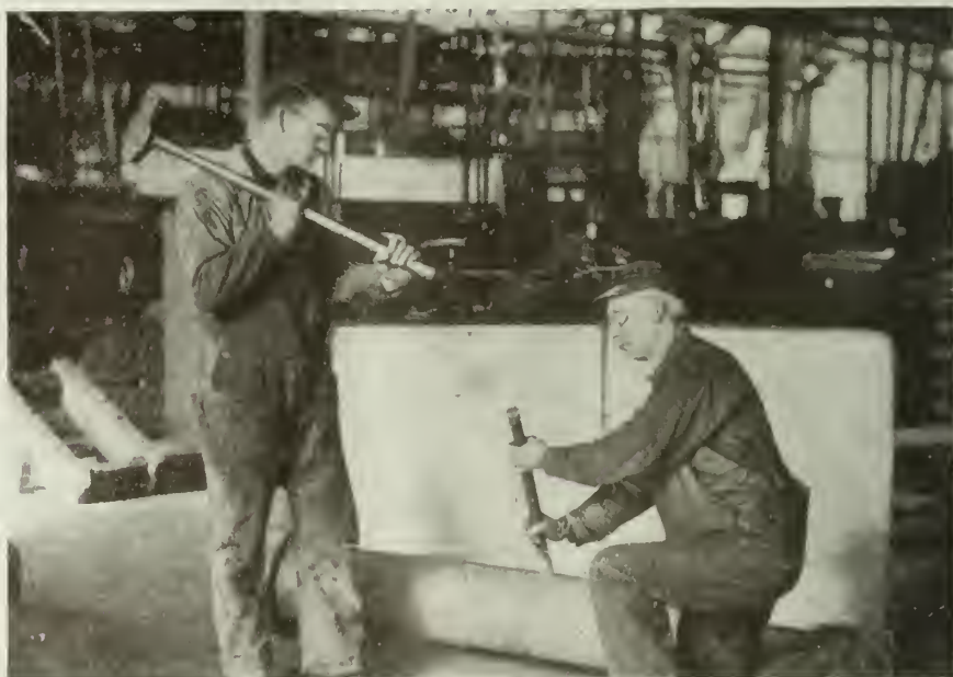
FIG. 37. WORKMEN CUTTING OUT RIVETS AND USING SHIELD. NOTE THAT GOGGLES ARE BEING WORN.
