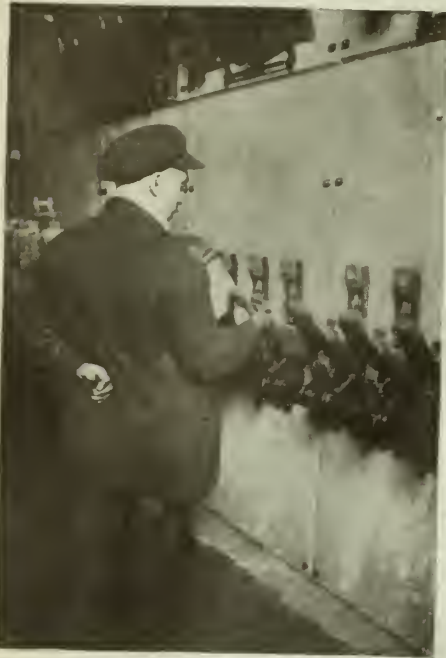
FIG. 40. SAFE WAY TO OPEN A SWITCH. USE ONE HAND AND KEEP OTHER BEHIND BACK.
