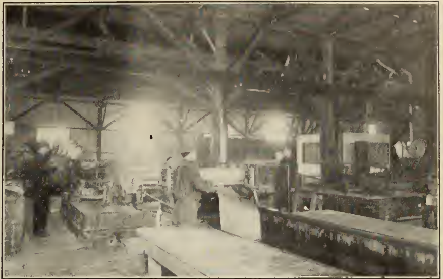
GALVANIZING MACHINE WITH FEED TANK.
