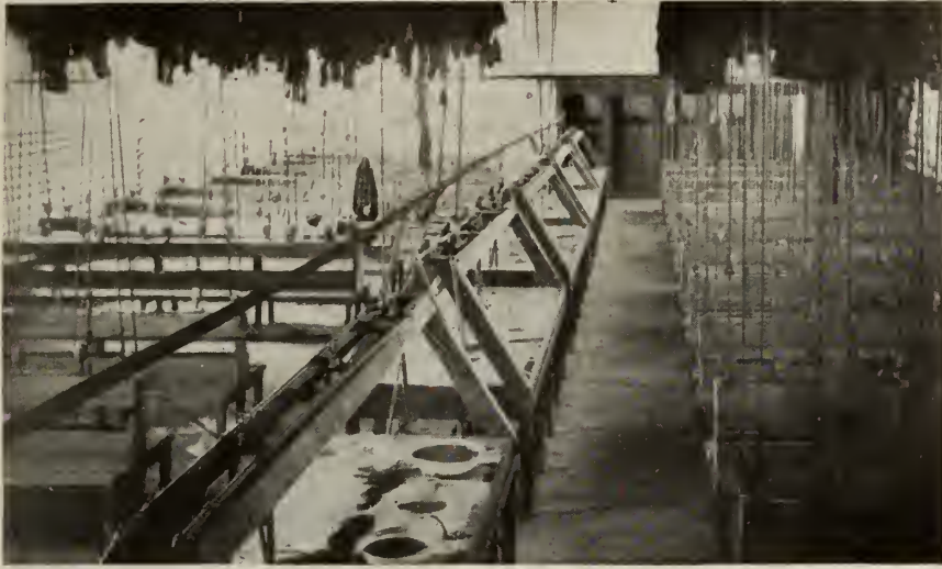
INTERIOR OF CHANGE HOUSE, SUBMARINE PLANT, WABANA, NFLD.
