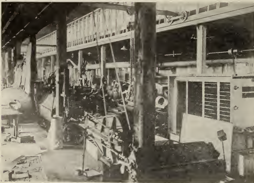
UPPER MACHINE SHOP, SHOWING GALVANIZED IRON WORK SECTION.
