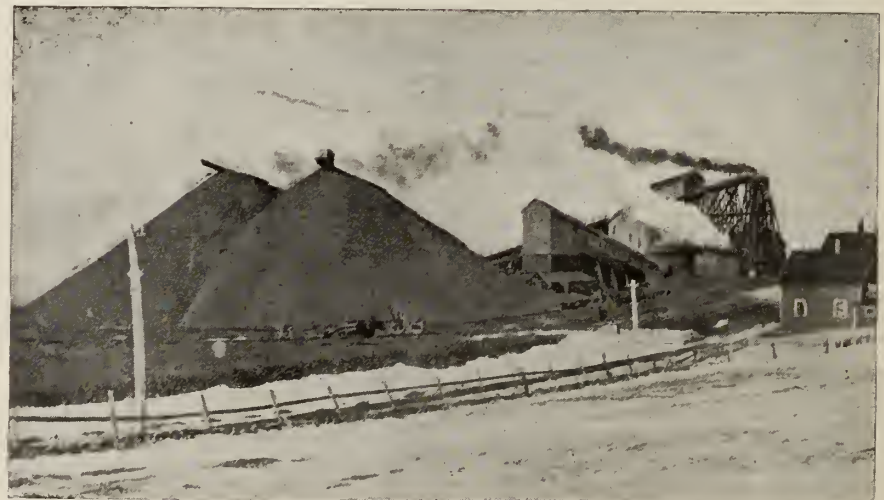
STOCK PILE AND DECK HEAD, SUBMARINE MINE, WABANA, NFLD.
