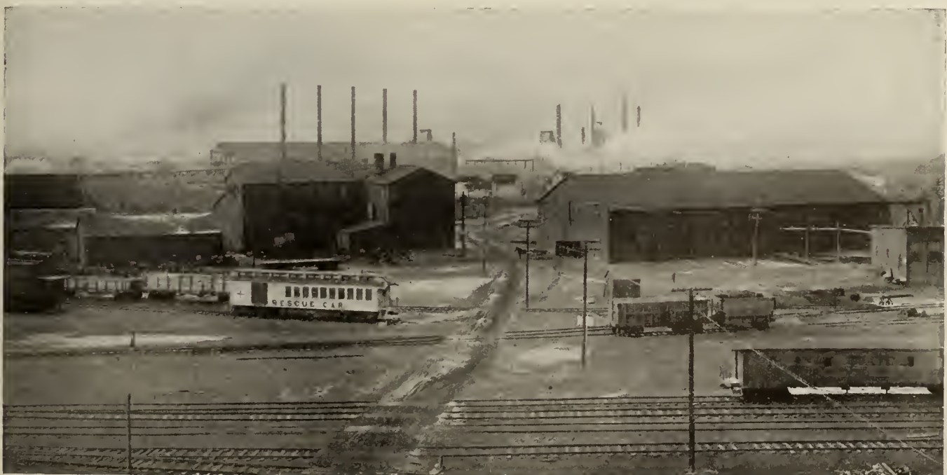
GENERAL VIEW FROM OFFICE OF STEEL PLANT AT SYDNEY MINES.
