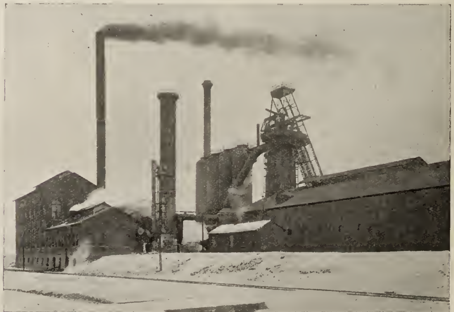
BLOWING ENGINE AND BOILER HOUSE, STOVES, BLAST FURNACE HOUSE AND EXTERIOR EQUIPMENT.
