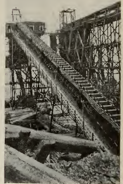
LOADING PIER, SHOWING CONVEYORS AT WABANA, NFLD.
