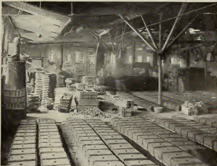
GENERAL VIEW OF MOULDING DEPARTMENT WITH MOULDS LAID OUT READY FOR POURING, JAMES SMART MFG. CO., BROCKVILLE.
