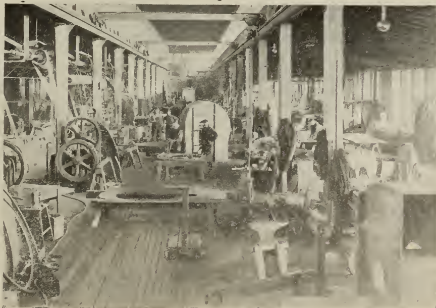
UPPER MACHINE SHOP. SHOWING FAN CASE ASSEMBLY SECTION.
