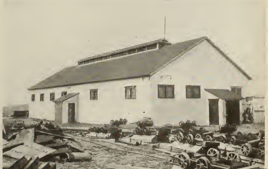
EXTERIOR OF CHANGE HOUSE, SUBMARINE PLANT, WABANA, NFLD.
