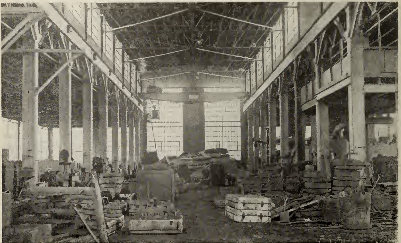
CENTRE BAY OF IRON FOUNDRY LOOKING EAST.
