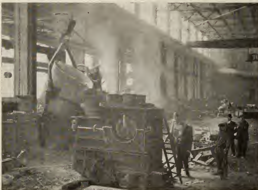
NEW GREY IRON FOUNDRY, SHOWING A LARGE LOCOMOTIVE CYLINDER BEING POURED.
