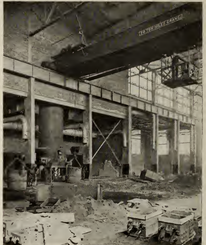
NEW GREY IRON FOUNDRY, SHOWING ONE OF THE CUPOLAS AND SPACES LEFT FOR ADDITIONAL UNITS.
