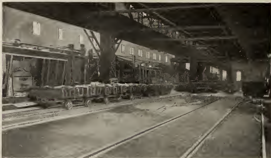
OPEN-HEARTH FURNACES AND CHARGING MACHINE, SYDNEY MINES.
