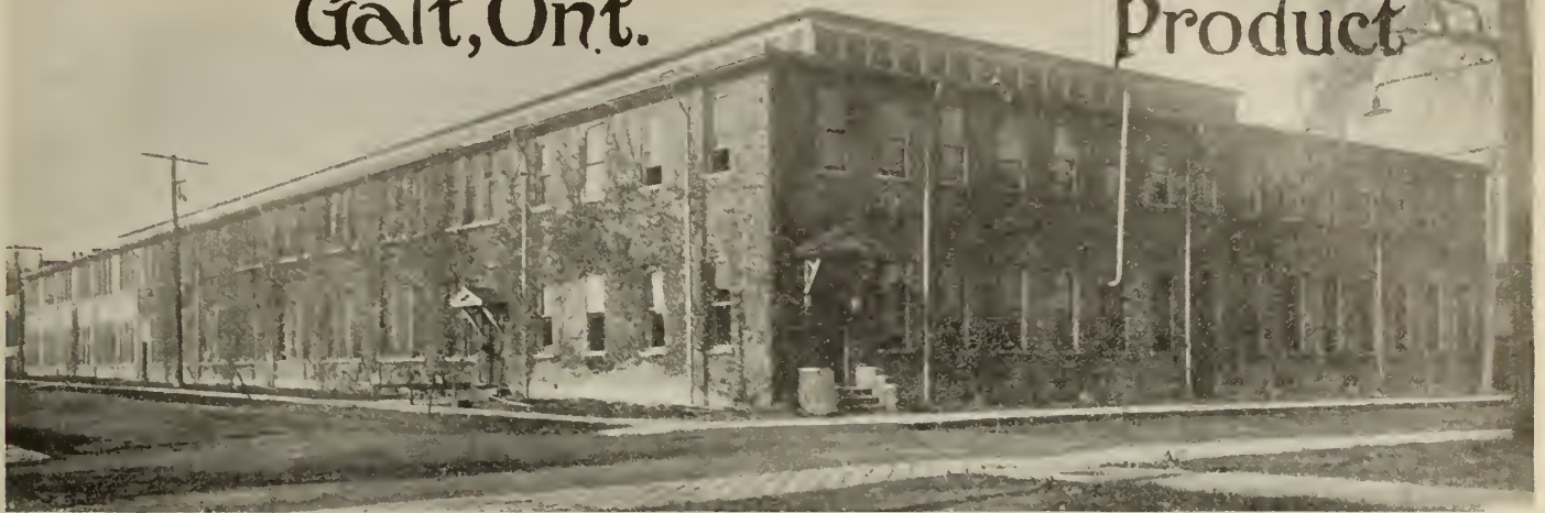
GENERAL VIEW SHOWING TWO FACES OF PLANT EXTERIOR. GENERAL OFFICES ON CORNER.
