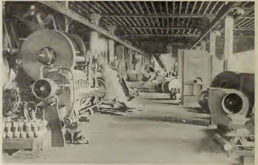
INTERIOR VIEW OF MACHINE SHOP, SHOWING FAN ERECTING FLOOR.
