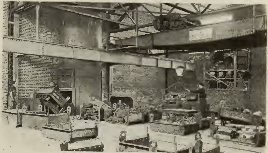
NEW GREY IRON FOUNDRY, SHOWING CUPOLA CHARGING FLOOR.
