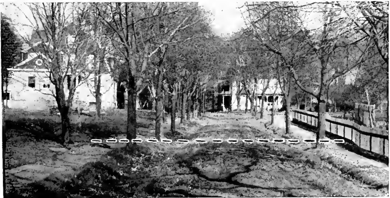
Fig. 25. Street grade raised two feet without changing sidewalk or injuring trees. Practicable only on a side street.
