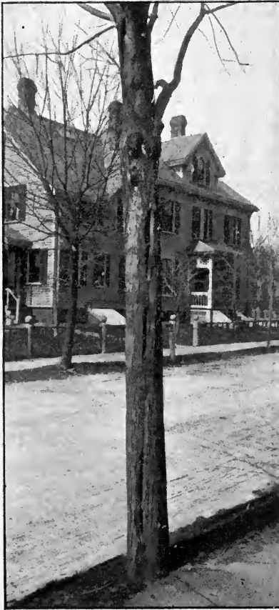
Fig. 10. Showing the effect of earth discharges through a tree, causing splitting of the trunk and destruction of limbs.
