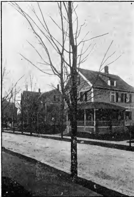
Fig. 11. Showing the effect of earth discharges through the tree, causing splitting of the trunk and destruction of limbs.
