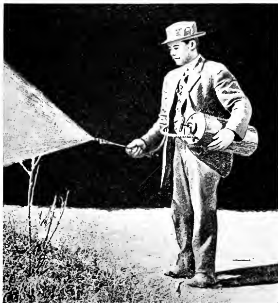
FIG. 221.—Compressed air sprayer, handy for garden use. (U.S.D.A.)
