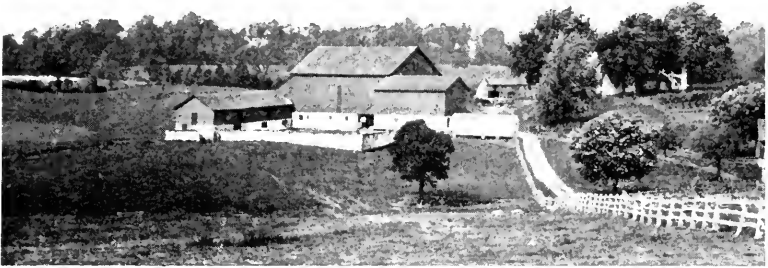
FIG. 267.—An ideal location for the farm buildings. The residence is among the trees on higher ground than the barns, which are also on a well-drained ridge. Note that all buildings are painted and kept up. (U.S.D.A.)
