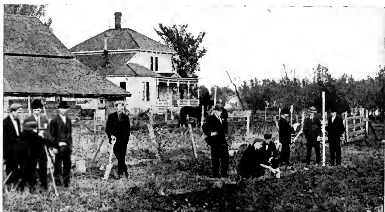
FIG. 92.—Students in a Minnesota high school doing the engineering work preliminary to tile drainage. (Minnesota Station).
