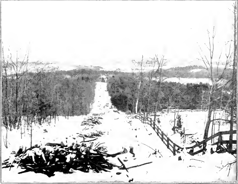
FIG. 19. — Fire line, Metropolitan Water Board reservation, Boylston.
