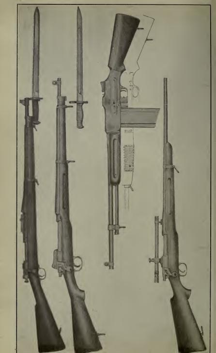
including the rod-bayonet, 8.937 pounds, and was 43.43 inches long. Until 1906 its cartridge gave a muzzle velocity of 2,200 to 2,300 foot seconds, used 42 to  $44\frac{1}{2}$  grains of nitro-glycerine smokeless powder, and a lead core, cupro-nickel covered, round nosed bullet weighing 220 grains.
