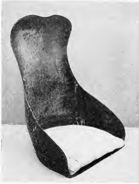
Fig. 213. Aviator's armored chair. Experimental model, American, 1918
