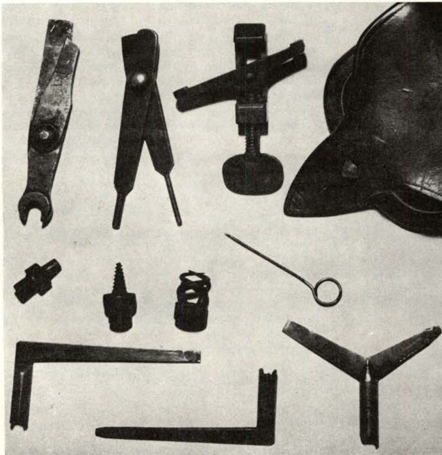
Accessories for CW guns were leather box for percussion caps, thumb-screw vise to cramp spring for stripping lock, pin punch for removing band springs and driving tumbler out of hammer, and combination two-blade screwdriver and nipple wrench. Extra nipple was often carried, together with screw fitting for ramrod to withdraw mis-fired bullet, and "worm" which held tow for wiping out bore. Wire loop is nipple pick to clear cap debris in case of misfire, while three angle tools are two Colt and one Whitney nipple wrenches.
