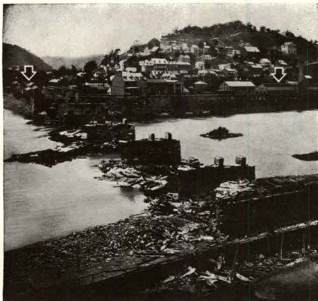
Photos like this one taken after Jackson's Raid reveal considerable damage to government arms factories there (rifle works, left; and rifle musket main armory, right arrow) but Confederates ran shops for several weeks making rifle muskets while remainder of stores and machinery were being moved South.
