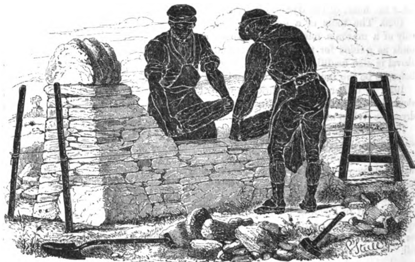
THE BUILDING A DRY-STONE DYKE.
