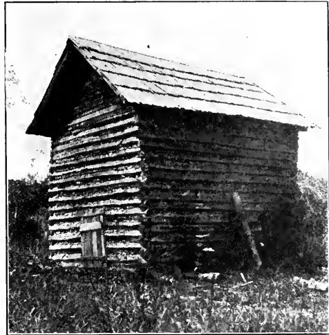
FLUE-CURING BARN, VIRGINIA.
