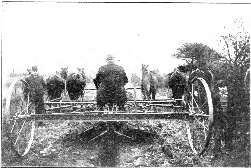
THE DITCHER IN OPERATION.
