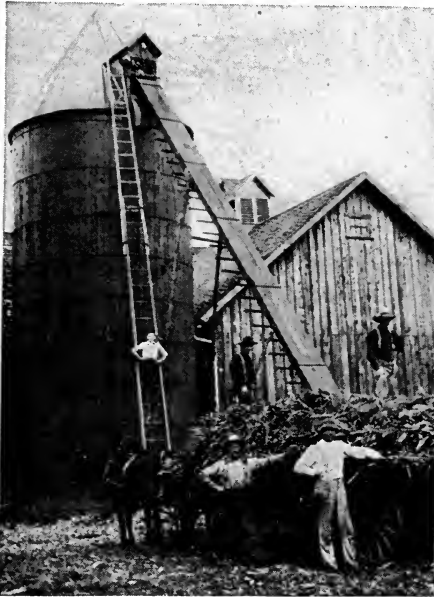
FIG. 80.—Silo filling. This silo is made from wooden staves and steel hoops, a structure common in the Eastern States. The ears and stalks are cut fine and carried up into the silo by the endless chain.
