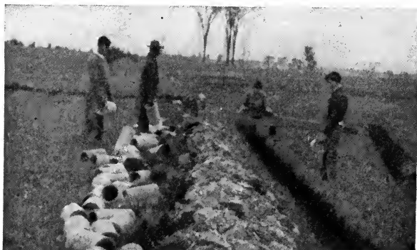
FIG. 38.—Ready to lay the six-inch drain tiles.
