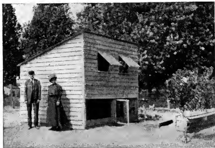
FIG. 195.—A colony house two stories high for laying hens. The nests and scratching litter are on the ground.
