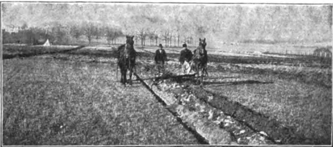
Fig. 163. The start and finish of tile draining.
