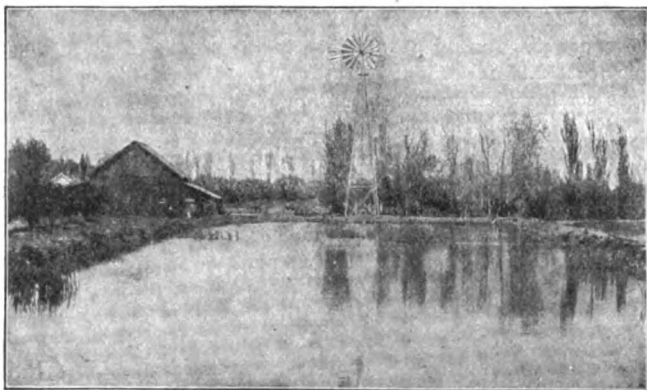
Fig. 76. Rectangular reservoir for windmill irrigation.
