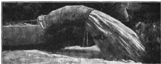
Fig. 68. Mouth of 8-inch discharge pipe 82 feet above Grand river, Grand Junction, Colorado.
