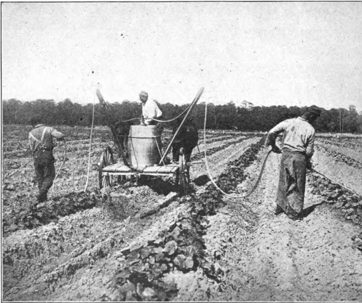
FIG. 109. Device for spraying cucumbers in the field (after Orton)
