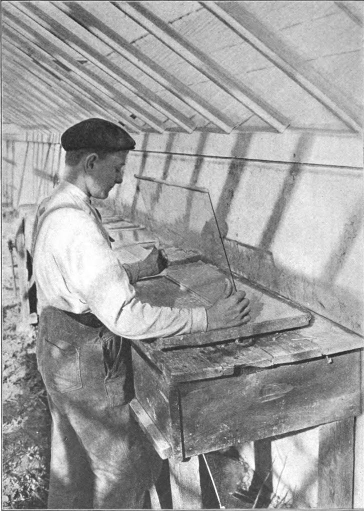
FIG. 19. Putting putty on the glass
