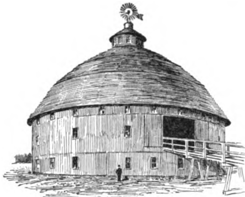
Fig. 181. A new type of circular barn erected in Indiana. No heavy timbers are employed in the construction. The bending system of framing is used.
