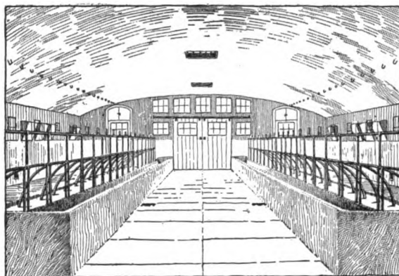
Fig. 320. The concrete trough runs the entire length of the building. The passageway between the double row of stanchions is about eight feet wide. All corners and right angles are finished with covers or in curves, so that dust does not collect or may be easily removed.
