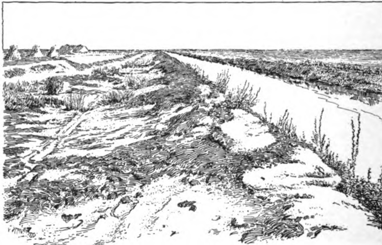
Fig. 688. Alkali appearing on ditch bank in Southern California.
