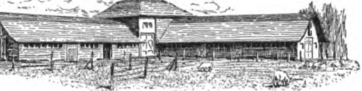
Fig. 179. A Wisconsin sheep-barn—rear elevation. It is of ordinary balloon frame construction, celled inside and outside, with shingle roof.
