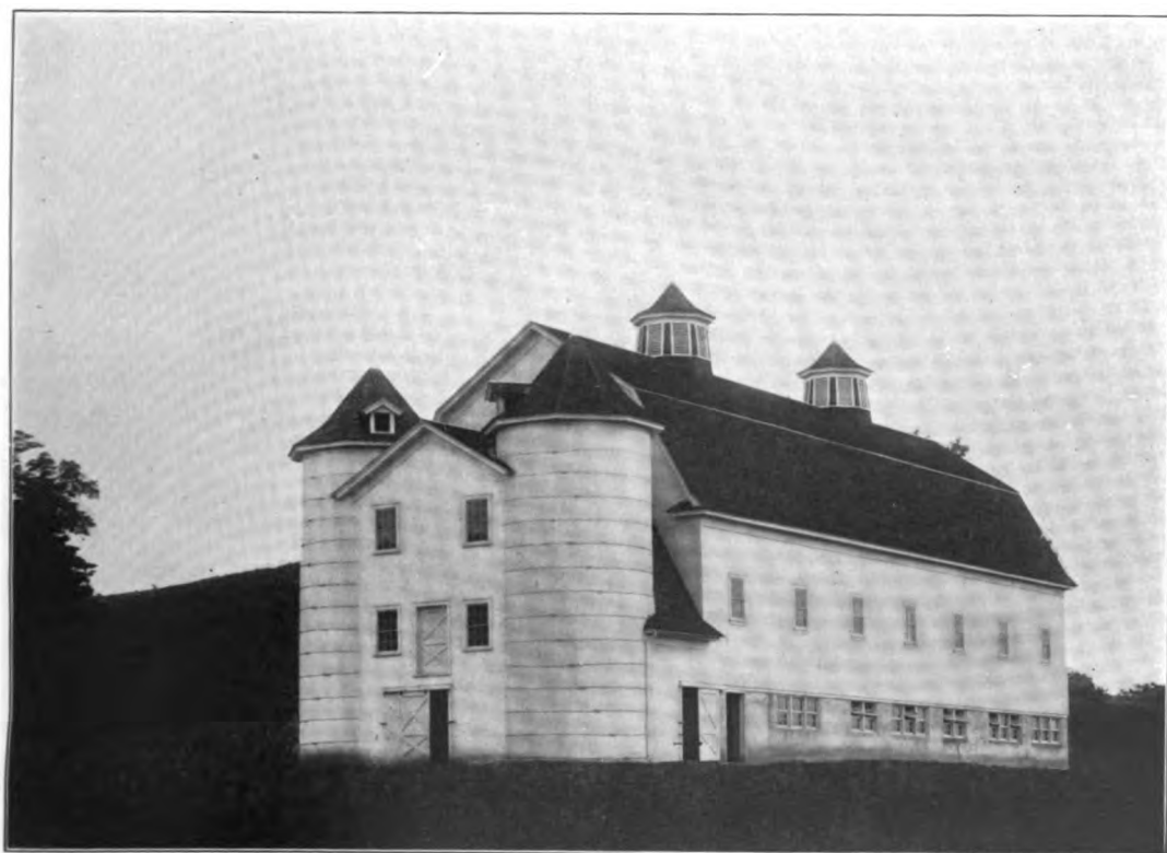
Plate XVI. An iron-frame trussed barn, said to be the first in America. The stable part is built of reinforced cement, the only wood being in the doors, window-frames and the front to the ventilators. The barn is sheathed with matched pine. F. E. Dawley, Fayetteville, New York.
