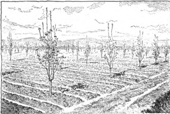
Fig. 211. Young orchard with two furrows on each side of rows for irrigation. View on Ashenfelter ranch, Montrose, Colorado.
