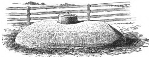
Fig. 417. Top of cemented cistern on a hill, before covering with earth.
