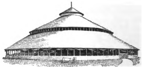
Fig. 182. Sanitary dairy-barn in the South. The open arrangement is well-adapted to the southern climates. Drop curtains furnish sufficient protection in inclement weather. (Fern Crest Dairy Farm, Sandersville, Ga.)
