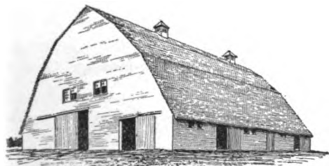
Fig. 180. A Kansas cattle-barn. There is ample storage for all the cattle that can get beneath the roof. The low roof deflects the winds harmlessly upward.
