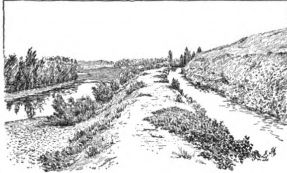
Fig. 687. Canal in gravelly river bluff, showing seepage of alkali in the killing of vegetation.
