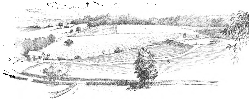
Fig. 273. The development of water power on a New York farm, by damming a small brook. The mill or shop is at E. The pond is at A, providing a head of 16 feet. The creek follows the line C; the other line, S, is a road. The mill is run by a 25-horse-power turbine. In the shop light sawing is done; and there are cider-press, bone-grinder, grindstone, feed-mill, and other power machines. A 7-horse-power wheel fed from the same flume runs a dynamo that supplies electric light for dwelling, yard and barns.
