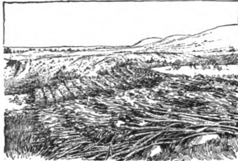
Fig. 582. A rock and brush irrigation dam in the Milk river valley, Montana.
