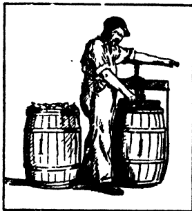
FIGURE 41.— Sweet potato barrels and device for pressing the heads into place.
