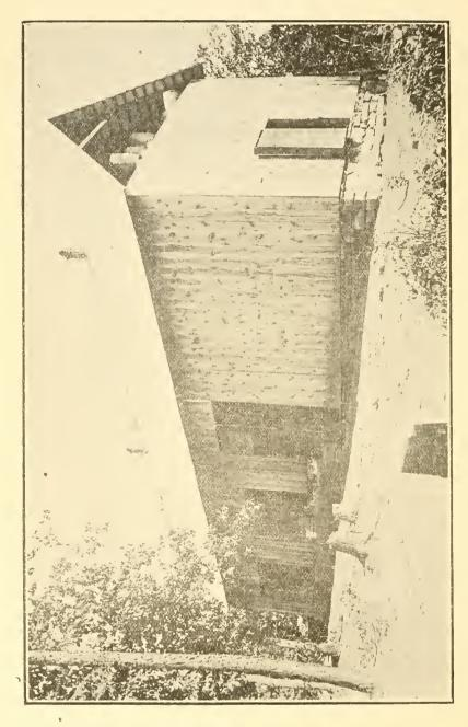
Potato House with walls and extension built later with 16-ft, walls and 4 tiers of bins, Size, 20x66.
