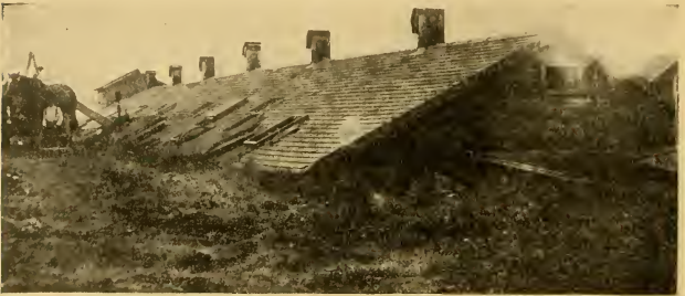
FIG. 126.—A good example of the type of storage house in use in the Red River Valley in Minnesota and North Dakota. This house has a water-tight roof with several openings in it to permit of spouting the potatoes into the storage bin. Sabin, Minn.
