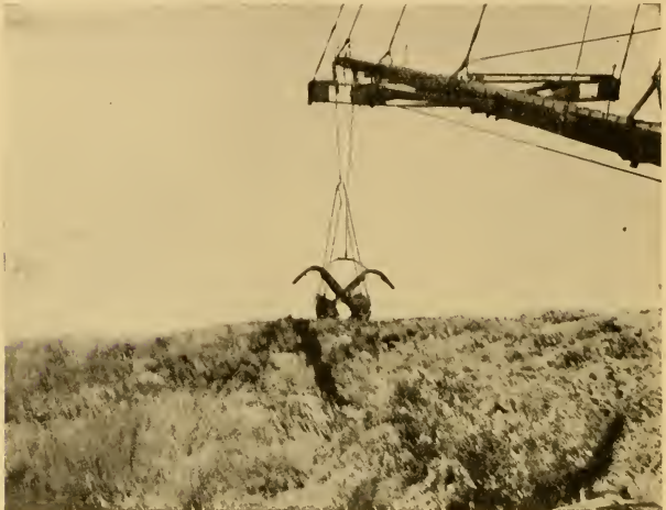
FIG. 54.—The first step in the reclamation of tule land is that of constructing a levee around a tract of land. The soil is scooped up by large scoops operated by a floating derrick.
