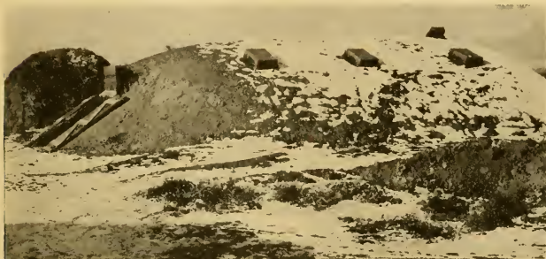
FIG. 119.—Side view of the house shown in Figure 118, with roof covered with straw and soil and ventilators capped.
