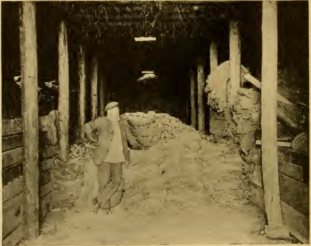
FIG. 128.—Method of filling a storage house in the Greeley district through openings in roof. Driveway partially filled by spouting potatoes through roof openings.
