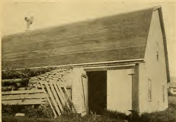
FIG. 131.—Exterior rear view of same house showing driveway entrance located in side of building at the rear end.
