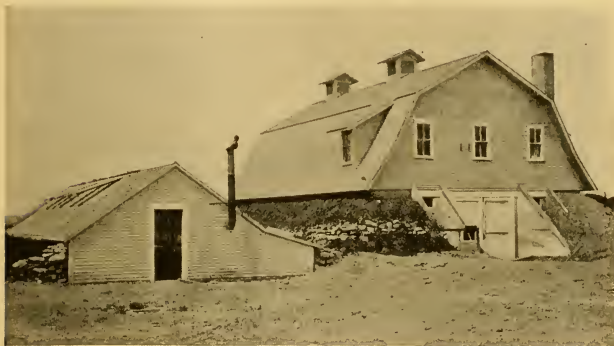
FIG. 133.—Potato storage house erected by the U. S. Dept. of Agriculture on Aroostook Farm, Presque Isle, Me. Note large roof ventilators or cupolas. Small greenhouse on left is used for starting the seed potatoes.
