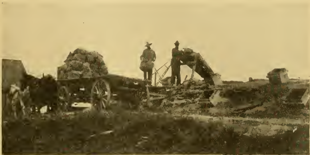
FIG. 127.—Spouting potatoes into storage cellar through chutes in the roof, in the Greeley, Col., district.
