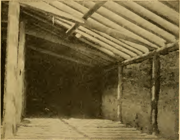
FIG. 121.—View showing earthen wall with plate supporting posts recessed into the bank. On the Sweet ranch, Carbondale, Col.
