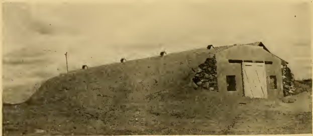
FIG. 122.—Partially sunken storage house with concrete side and end walls. Jerome, Idaho.
