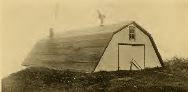
FIG. 130.—Exterior front view of a Maine type of storage house. This particular house is an exception to the general rule in that it is provided with a roof ventilator.
