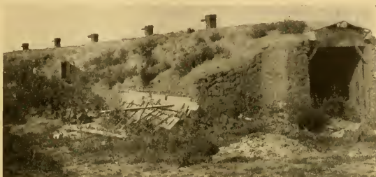
FIG. 114.—A good example of a sod-walled potato storage house near Greeley, Col. This house is provided with ridge and side ventilators.
