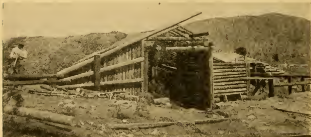
FIG. 111.—Exterior view of a large potato storage cellar in process of construction on the Sweet ranch, Carbondale, Colorado, showing construction of vestibule entrance and the covering of roof with straw.
