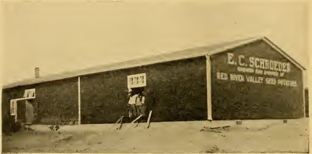
FIG. 124.—A typical Red River Valley potato warehouse with a deep cement-walled basement cellar. Glyndon, Minn.
