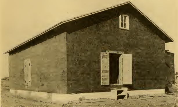
FIG. 129.—A good example of an insulated wooden structure used for the storage of potatoes in some localities in Michigan.
