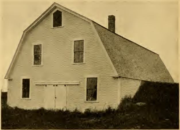
FIG. 132.—The more common type of the better class of Maine potato storage houses, with rear end driveway.
