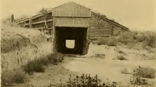
FIG. 113.—Completed structure showing cribbed vestibule on the Sweet ranch, Carbondale, Col.
