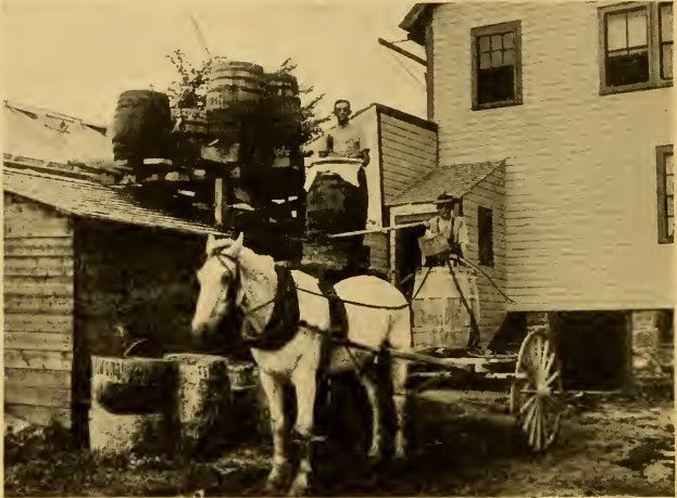
FIG. 185.—Spray mixing platform at the Vermont Experiment Station showing operation of filling spray barrel. Barrels in rear of upper platform contain the stock solutions, those in the front are the dilution barrels while the one with the strainer is the mixing barrel.
