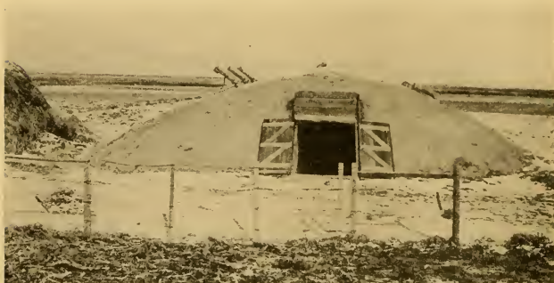
FIG. 120.—A frontal view of the completed potato storage house (Fig. 118) showing driveway entrance and ventilator caps raised on left side.
